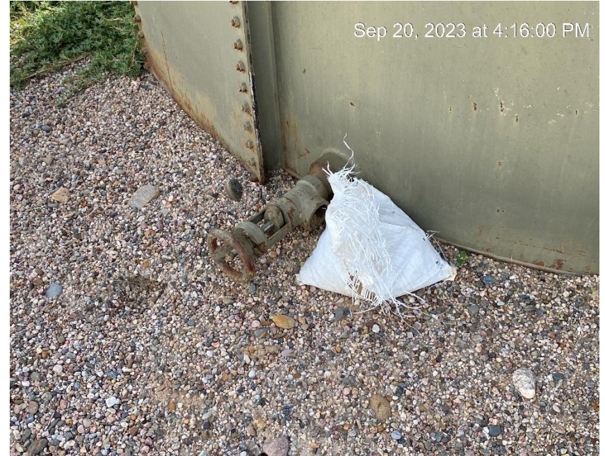
Debris. Open end tank valve
