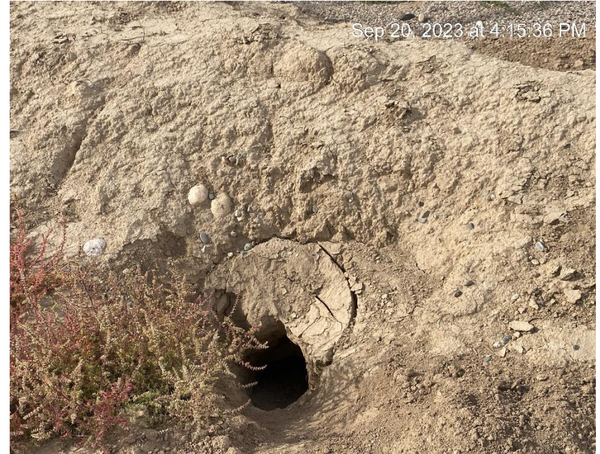
Tank berm burrow
