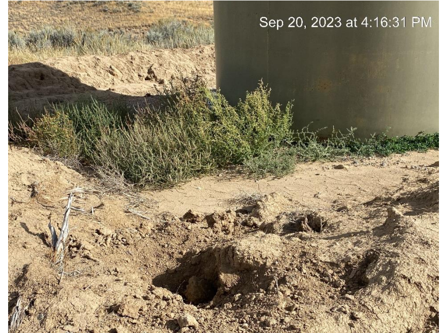
Weeds. Insufficient tank berm
