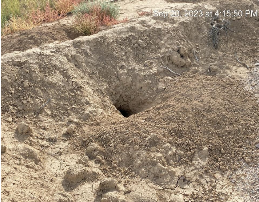
Insufficient tank berm
