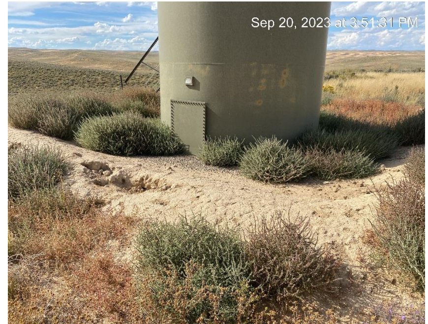
Weeds. Tank berm insufficient
