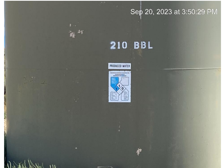
Tank labels insufficient
