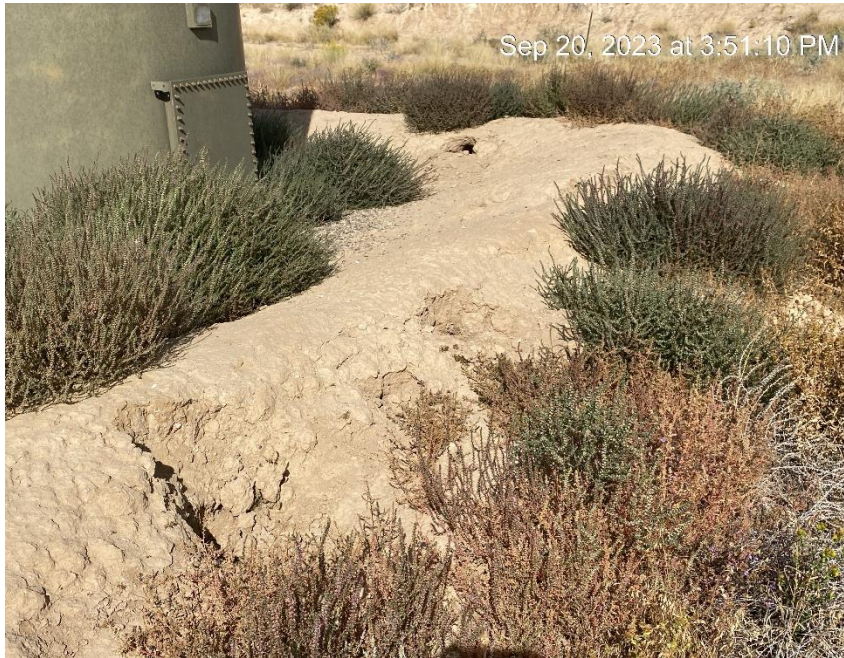
Weeds. Tank berm insufficient
