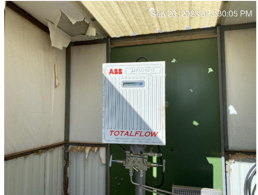
No visible display of gas calibration
