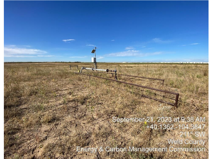
Gas Meter Run & Overgrown Vegetation
