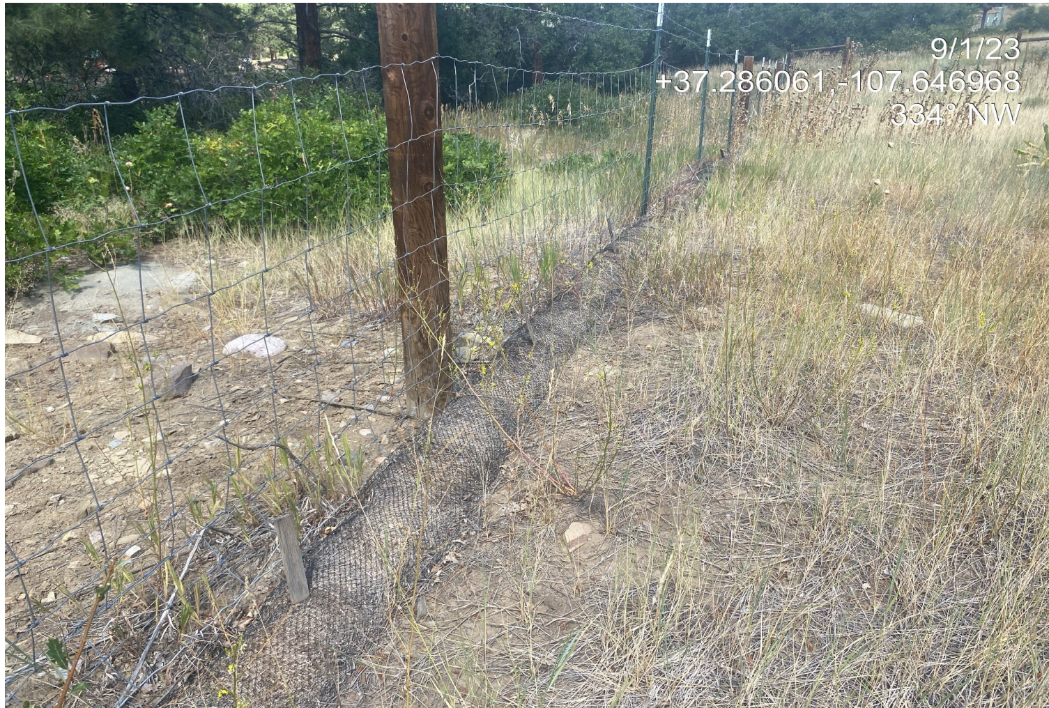
Photo 3. View of the southern edge of the disturbance. Several wooden stakes remain and wattle stormwater BMPs that need to be removed.
