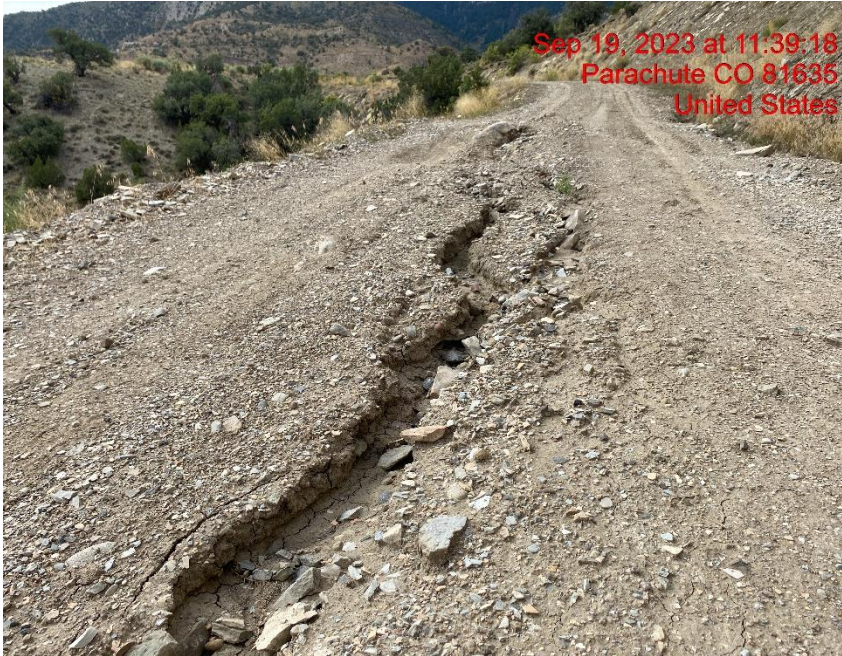
Rill Erosion Cutting Through Access Road – Photo #06481
