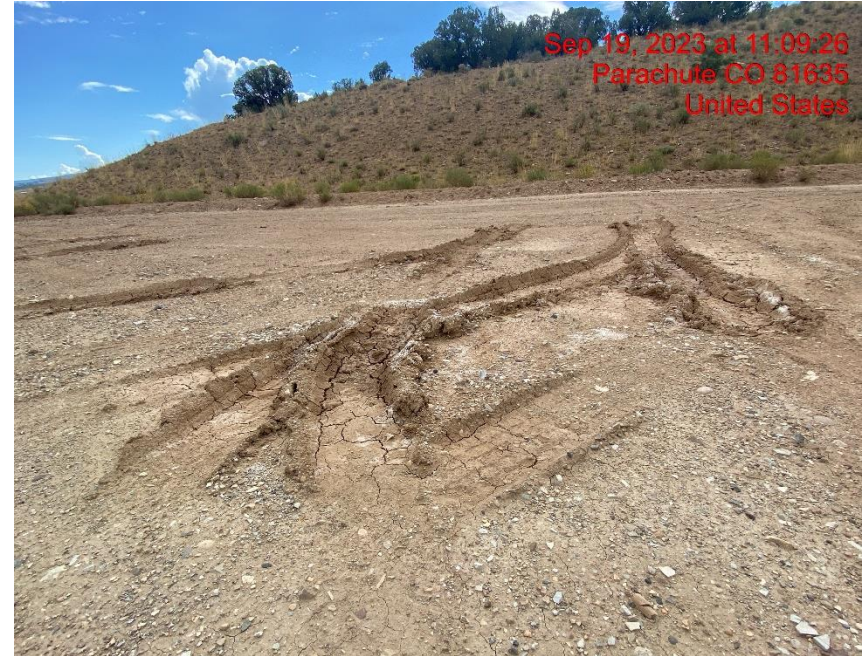
Location Lacks Stabilization – Photo #06470
