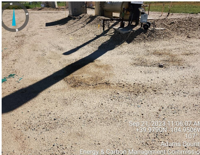
Photo 7 stained soil out side equipment berm
