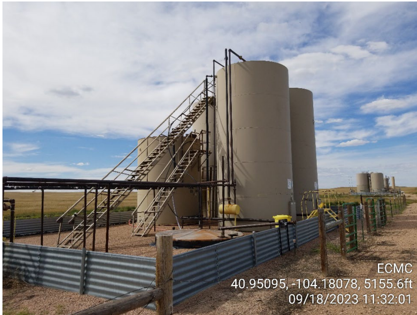
Photo 3 – Tank Battery
