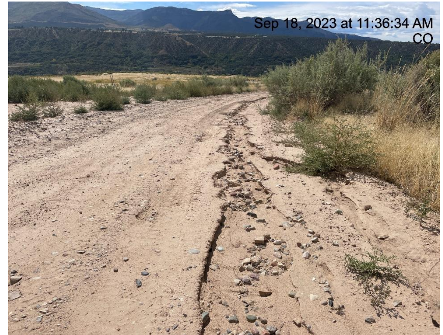
Photo # 9621 Erosion & transport of sediment on access road
