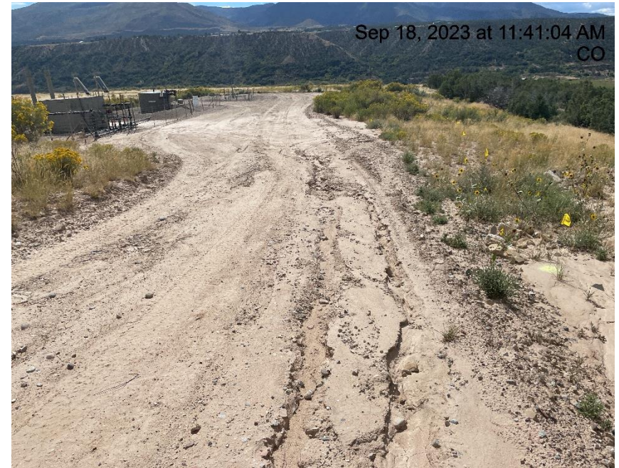
Photo # 9644 Erosion & transport of sediment on access road & then onto location & into vegetated areas
