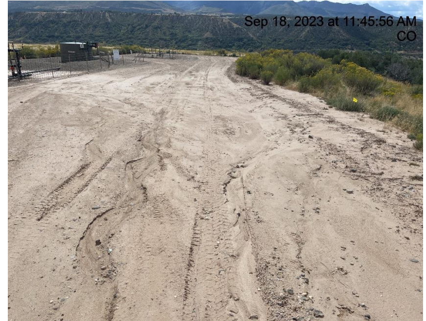
Photo # 9669 Sediment transported from access road onto location & into vegetated areas
