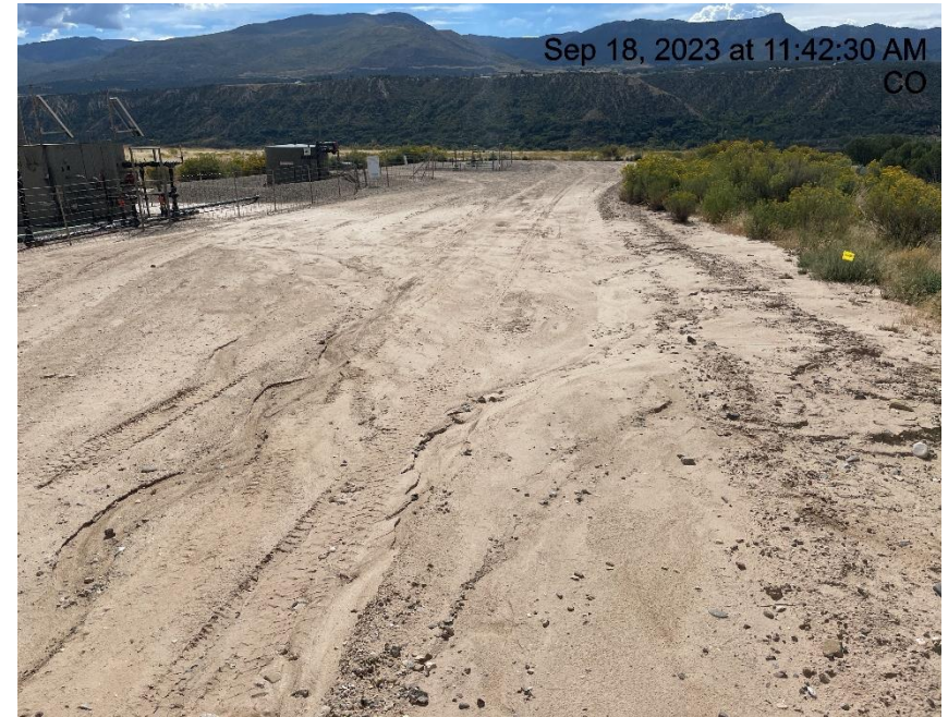
Photo # 9648 Erosion & transport of sediment on access road & then onto location & into vegetated areas
