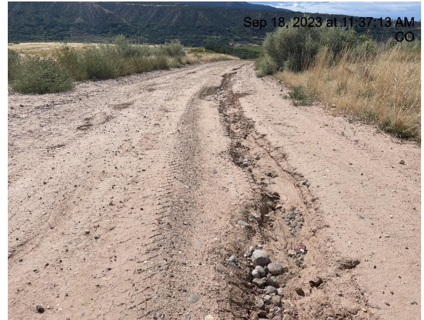
Photo # 9623 Erosion & transport of sediment on access road
