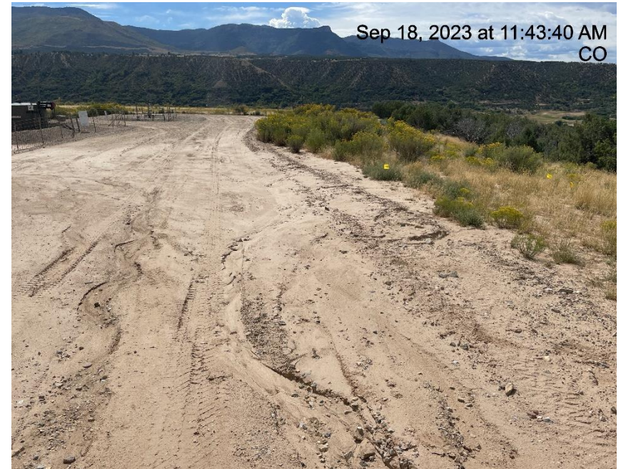
Photo # 9655 Erosion & transport of sediment on access road & then onto location & into vegetated areas
