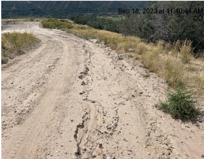
Photo # 9641 Erosion & transport of sediment on access road & then onto location & into vegetated areas
