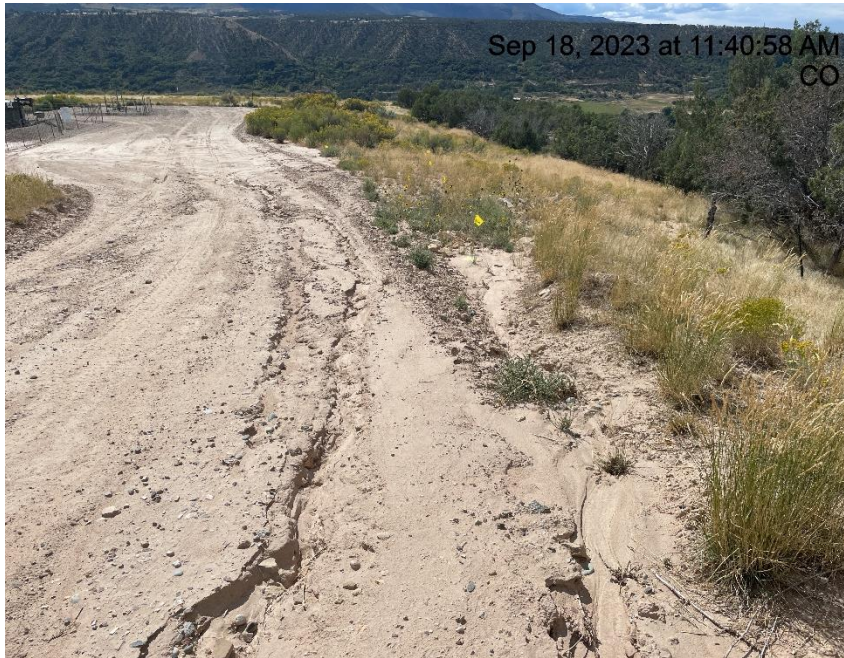
Photo # 9643 Erosion & transport of sediment on access road & then onto location & into vegetated areas
