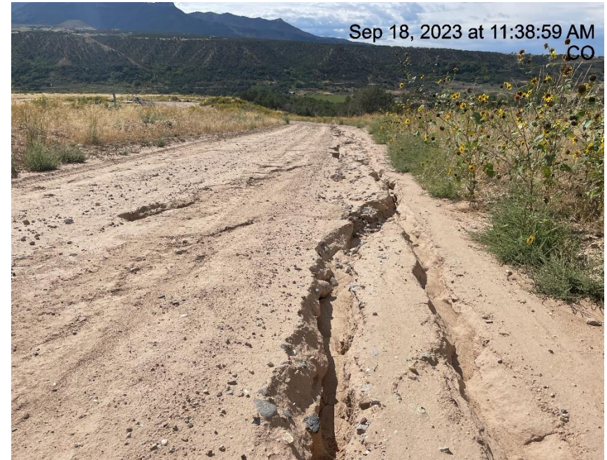
Photo # 9630 Erosion & transport of sediment on access road
