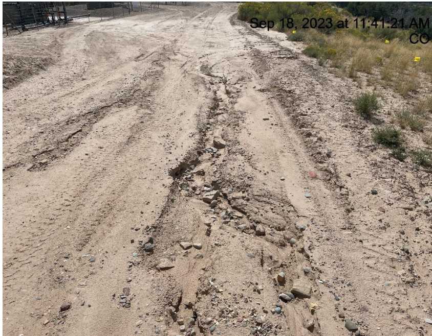
Photo # 9645 Erosion & transport of sediment on access road & then onto location & into vegetated areas
