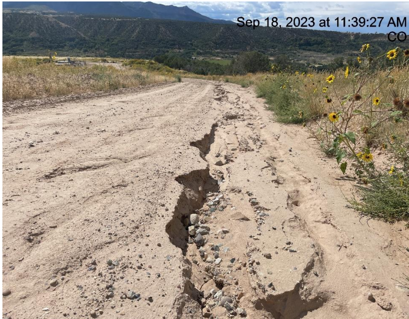
Photo # 9634 Erosion & transport of sediment on access road
