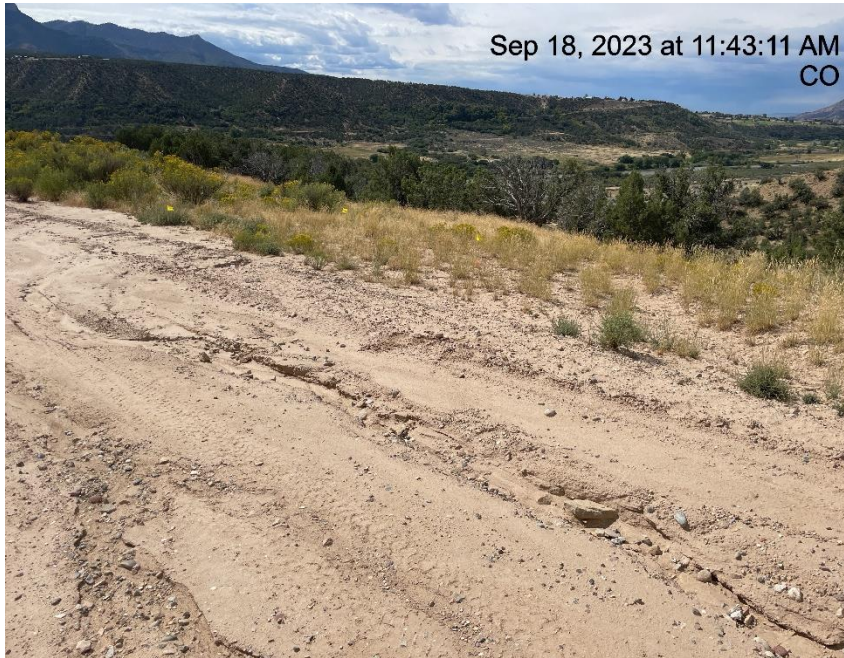
Photo # 9652 Erosion & transport of sediment on access road & then onto location & into vegetated areas
