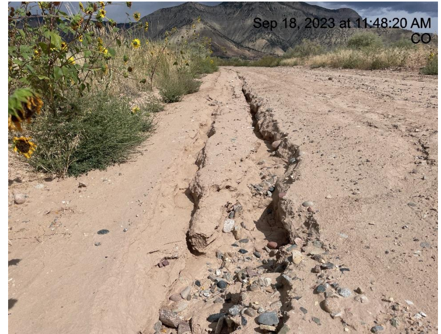
Photo # 9683 Erosion & transport of sediment on access road
