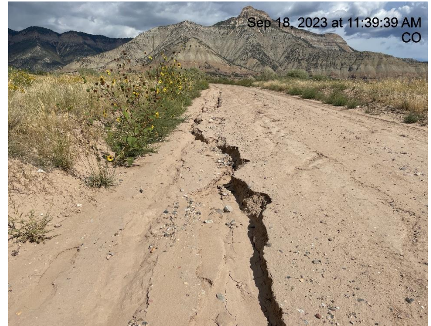
Photo # 9635 Erosion & transport of sediment on access road
