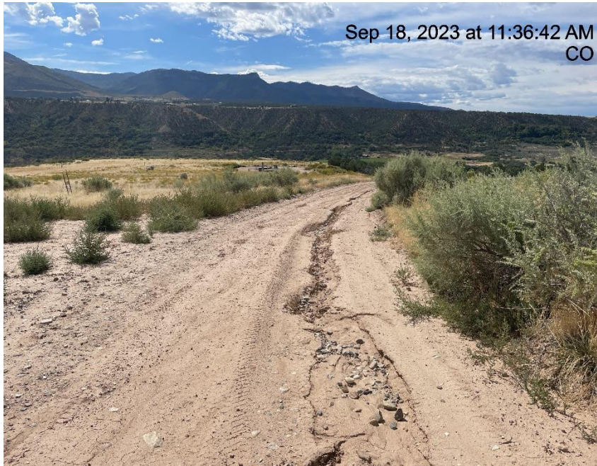
Photo # 9622 Erosion & transport of sediment on access road
