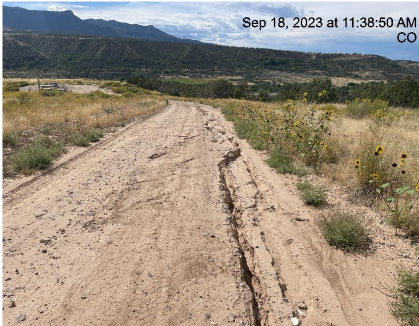
Photo # 9629 Erosion & transport of sediment on access road
