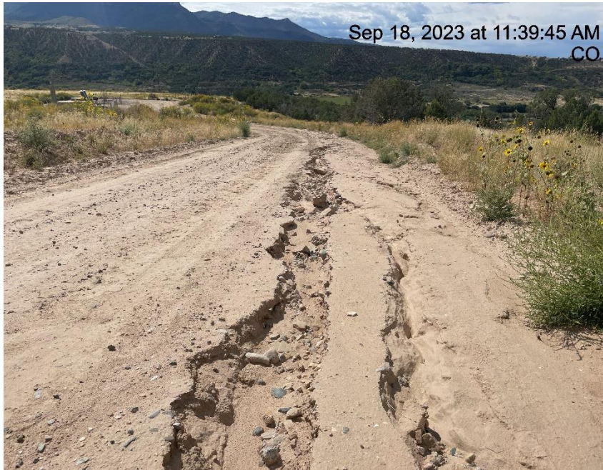
Photo # 9636 Erosion & transport of sediment on access road
