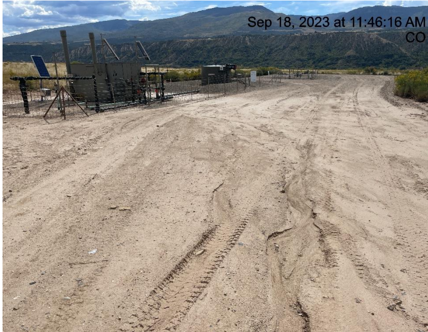
Photo # 9668 Sediment transported from access road onto location & into vegetated areas
