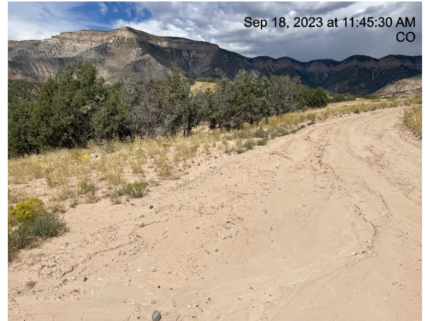
Photo # 9665 Erosion & transport of sediment on access road & then onto location & into vegetated areas
