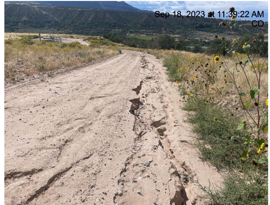
Photo # 9633 Erosion & transport of sediment on access road
