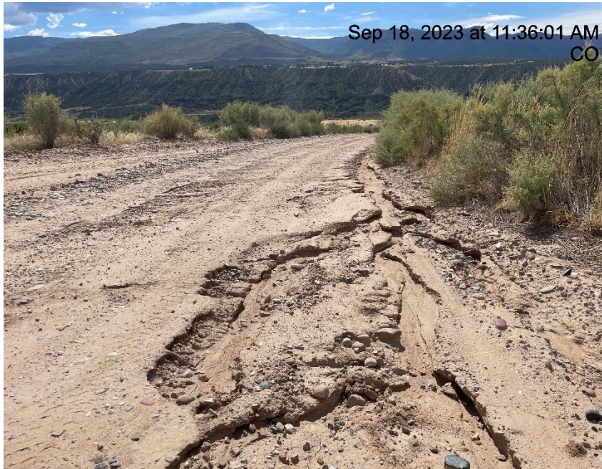
Photo # 9620 Erosion & transport of sediment on access road
