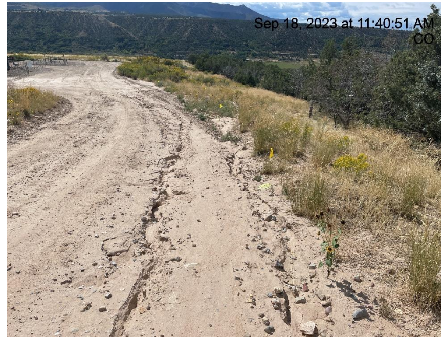
Photo # 9642 Erosion & transport of sediment on access road & then onto location & into vegetated areas
