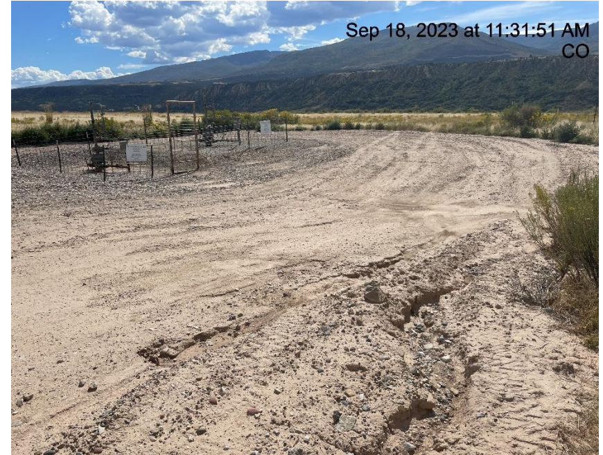
Photo # 9618 Erosion & transport of sediment on location
