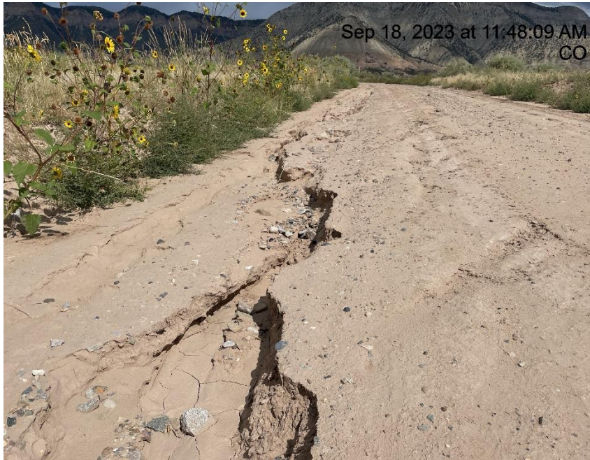
Photo # 9682 Erosion & transport of sediment on access road
