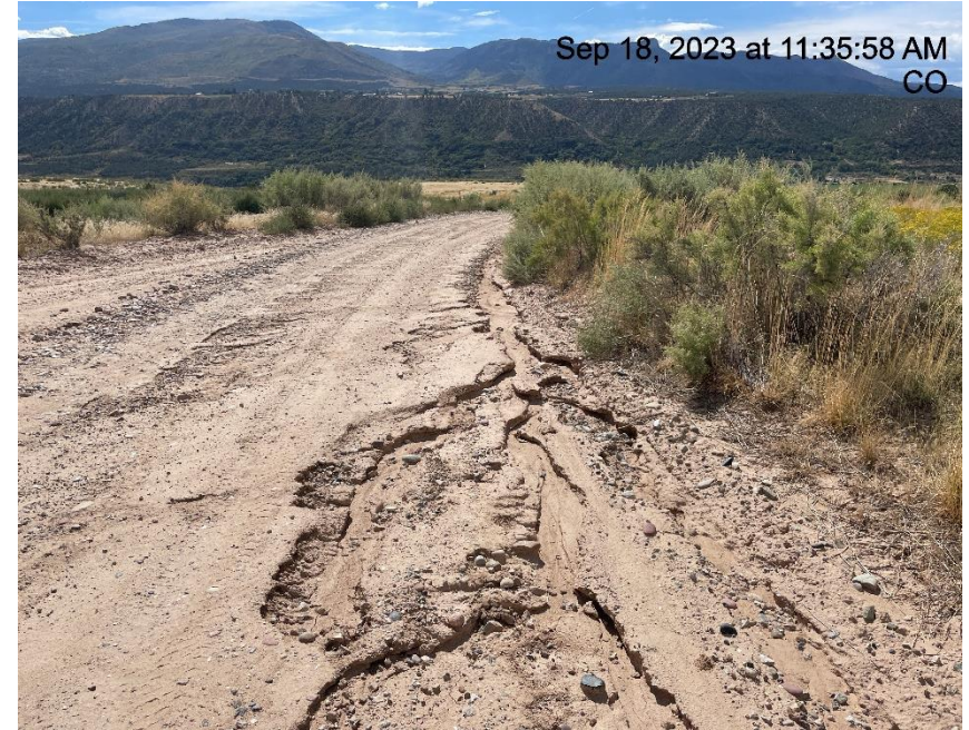
Photo # 9619 Erosion & transport of sediment on access road
