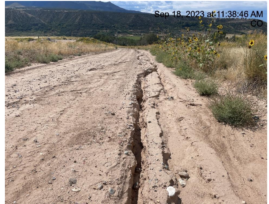
Photo # 9628 Erosion & transport of sediment on access road
