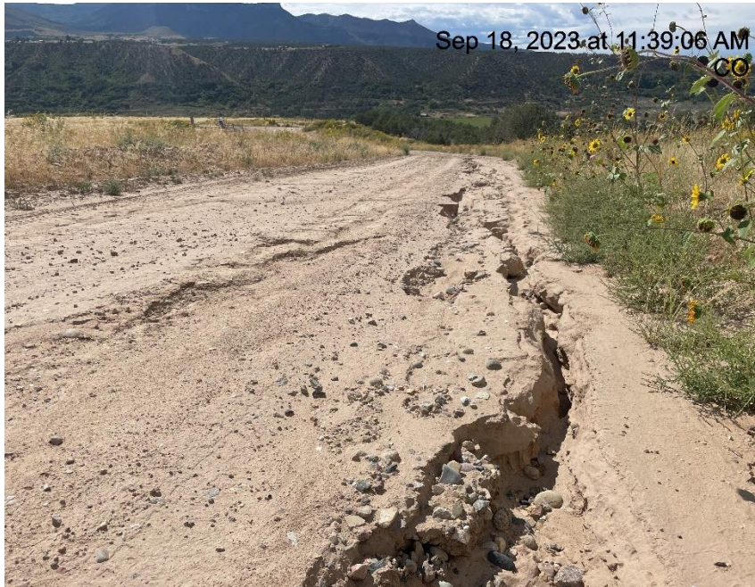
Photo # 9631 Erosion & transport of sediment on access road
