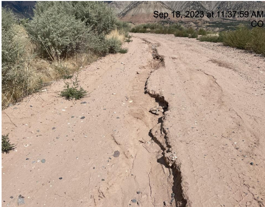
Photo # 9626 Erosion & transport of sediment on access road
