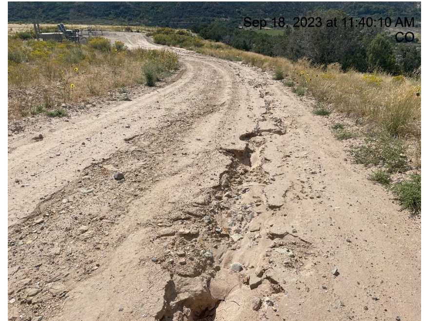
Photo # 9638 Erosion & transport of sediment on access road
