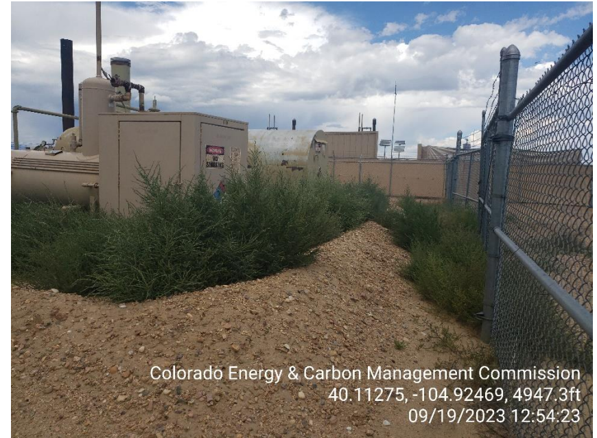
Photo 10 Undesirable vegetation growing tall around the horizontal Heater Treater and Horizontal Heated Separator.
