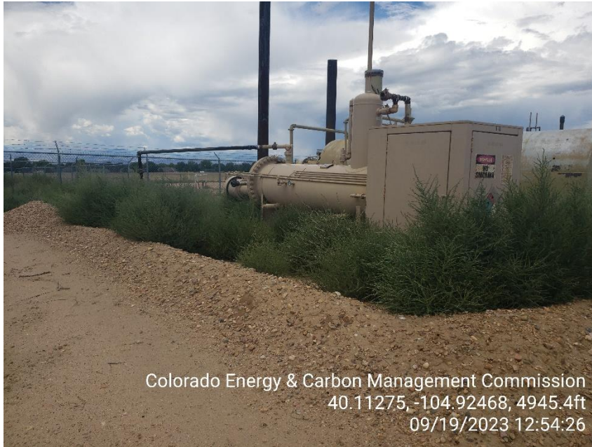
Photo 11 Undesirable vegetation growing tall around the horizontal Heater Treater and Horizontal Heated Separator.
