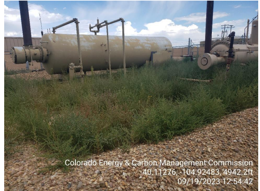
Photo 12 Undesirable vegetation growing tall around the horizontal Heater Treater and Horizontal Heated Separator.
