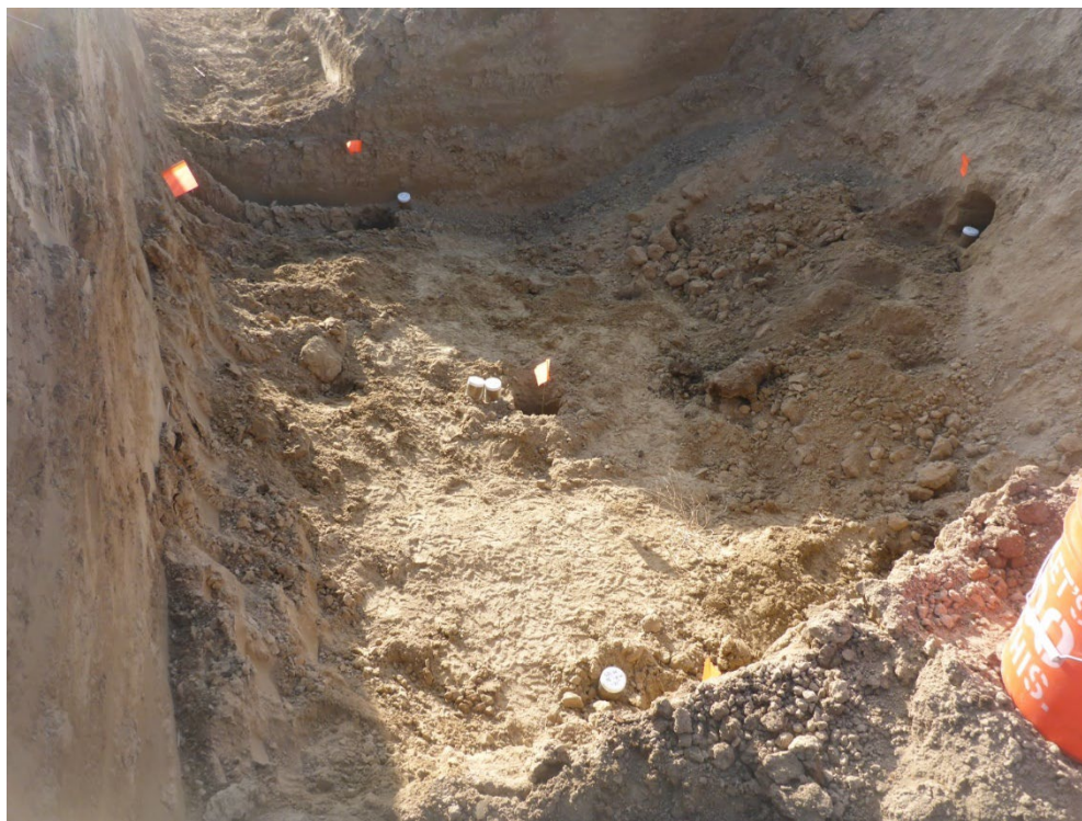
Sample Point G1c (Looking West) Excavation of contaminated soils and sampled for closure.
