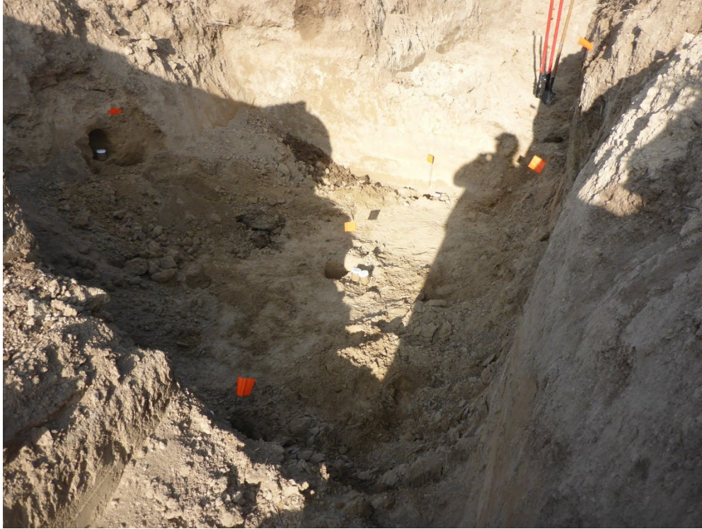
Sample Point G1b (excavation of contaminated soil and samples G1b2 for closure)
