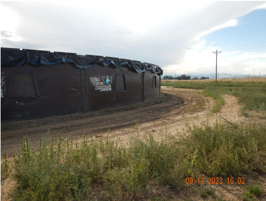
Photo 1. Photo taken from the northeastern interim reclamation area, facing West. Photo illustrates a MLVT has been constructed for subsequent well operations with heavy equipment. Operator has graded and disturbed the area for the purposes of constructing a MLVT.
