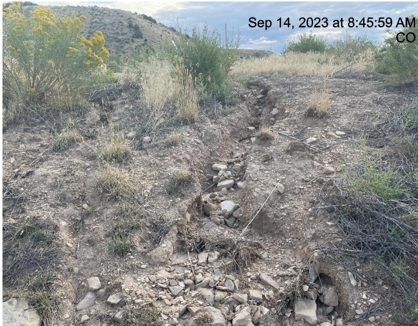
Photo # 9147 Erosion & transport of sediment off location into a vegetated area/choking off vegetation/insufficient BMP's .
