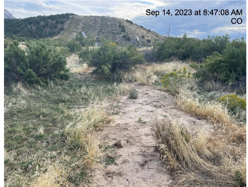
Photo # 9155 Erosion & transport of sediment off location into a vegetated area/choking off vegetation/insufficient BMP's .
