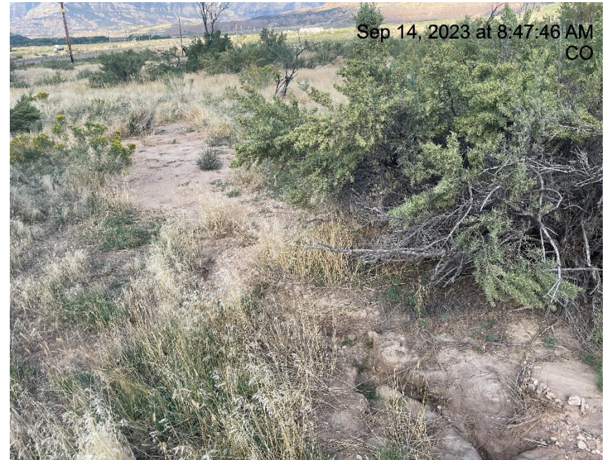
Photo # 9161 Erosion & transport of sediment off location into a vegetated area/choking off vegetation/insufficient BMP's .
