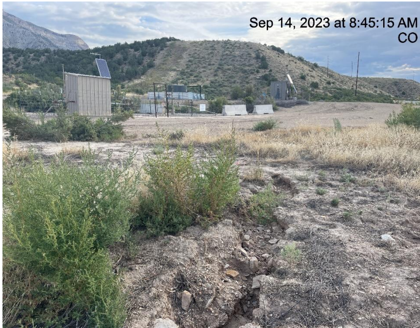
Photo # 9140 Erosion & transport of sediment off location into a vegetated area/choking off vegetation/insufficient BMP's .
