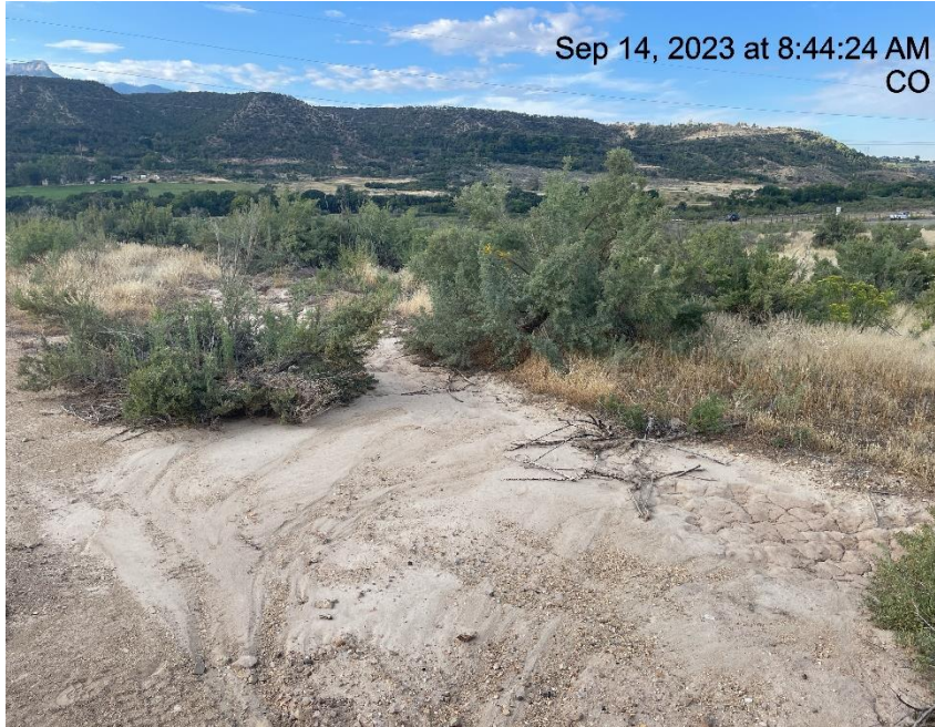
Photo # 9134 Erosion & transport of sediment off location into a vegetated area/choking off vegetation/insufficient BMP's .
