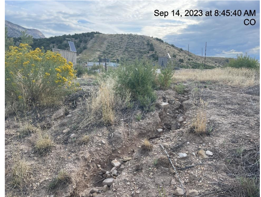
Photo # 9143 Erosion & transport of sediment off location into a vegetated area/choking off vegetation/insufficient BMP's .
