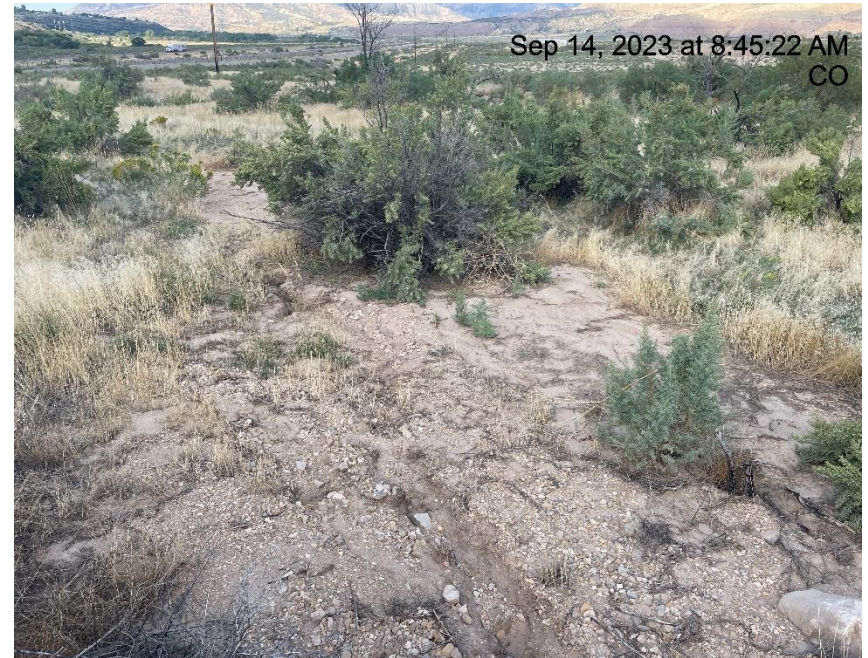
Photo # 9141 Erosion & transport of sediment off location into a vegetated area/choking off vegetation/insufficient BMP's .
