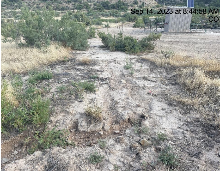
Photo # 9138 Erosion & transport of sediment off location into a vegetated area/choking off vegetation/insufficient BMP's .
