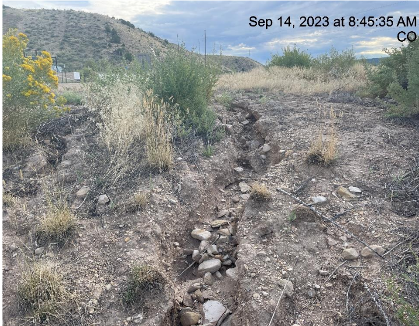
Photo # 9142 Erosion & transport of sediment off location into a vegetated area/choking off vegetation/insufficient BMP's .
