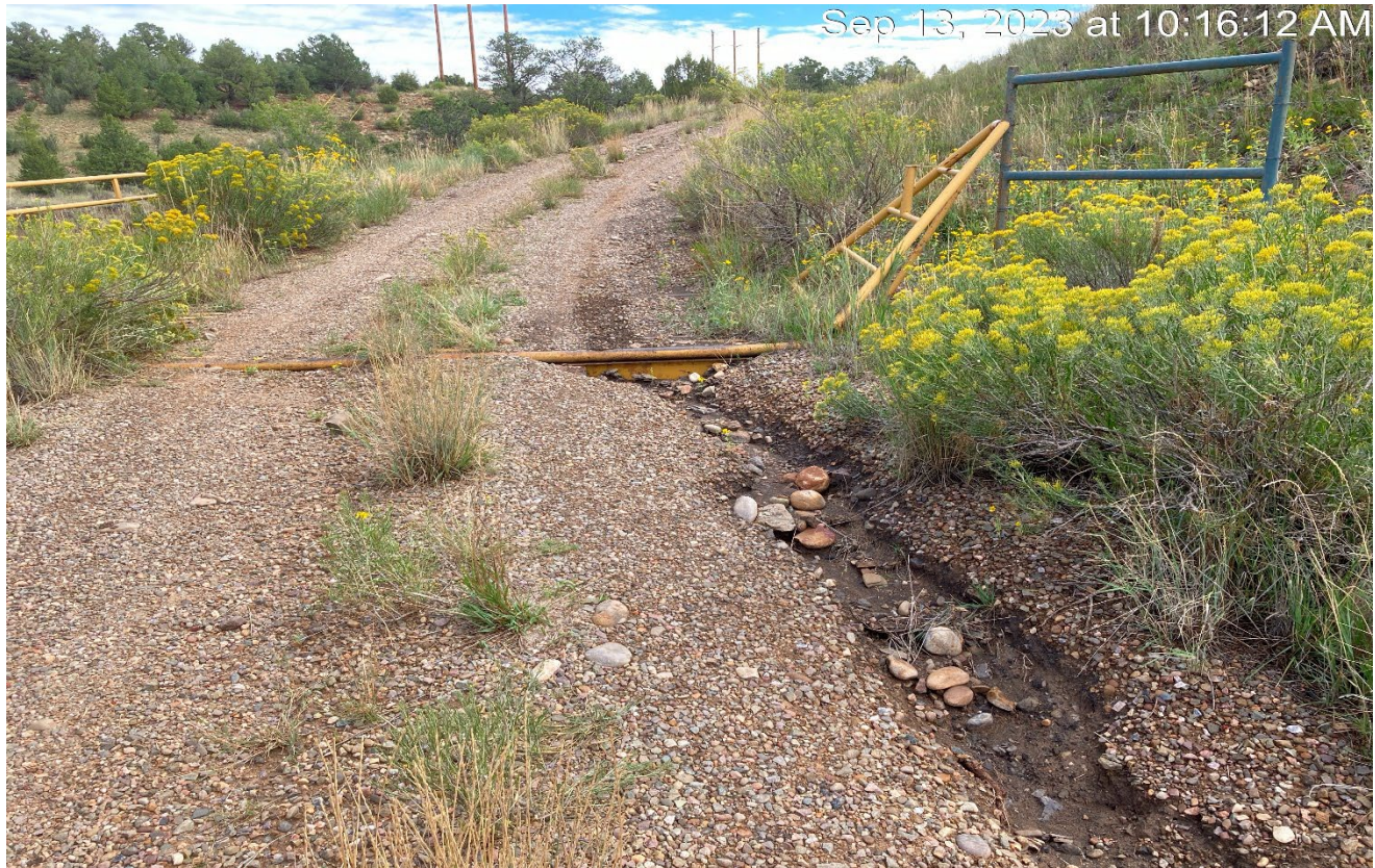
Photo 1. Facing east along the access road. The cattle guard is filled in with sediment and erosion is occurring at this area.
