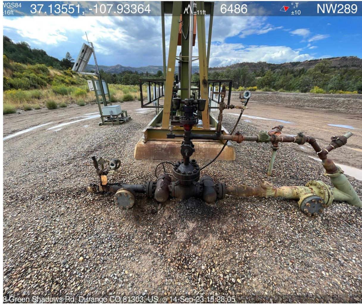
Photo #3 View of impacted material on ground at wellhead.
