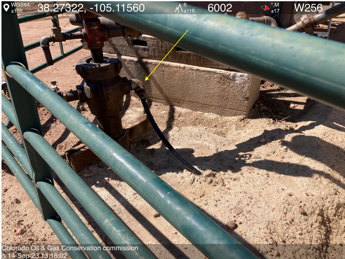
PHOTO 9: T-C ANNULUS PLUMBED TO CRUDE OIL TANK BATTERY.
