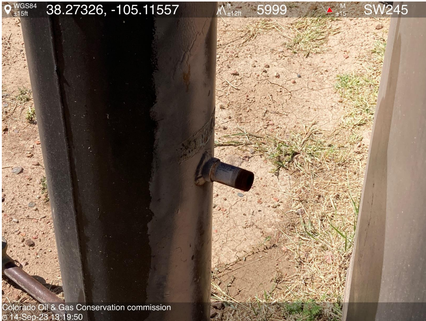
PHOTO 12: SEPARATOR IN LINE WITH 1" T-C ANNULUS SUPPLY LINE TO TANK BATTERY IS OPEN TO ATMOSPHERE. Tanks will function as sealed and ventless with gas released only through a vapor control system or properly sized pressure relief valve. per Rule 608.a.(9). 24 HOURS TO ADDRESS THIS CORRECTIVE ACTION.
