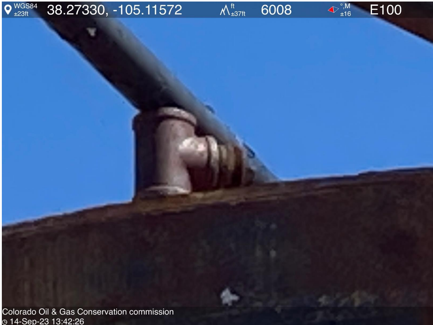
PHOTO 8: NO PRESSURE RELIEF VALVE. Tanks will function as sealed and ventless with gas released only through a vapor control system or properly sized pressure relief valve. per Rule 608.a.(9). 24 HOURS TO INSTALL PRESSURE RELIEF VALVE.
