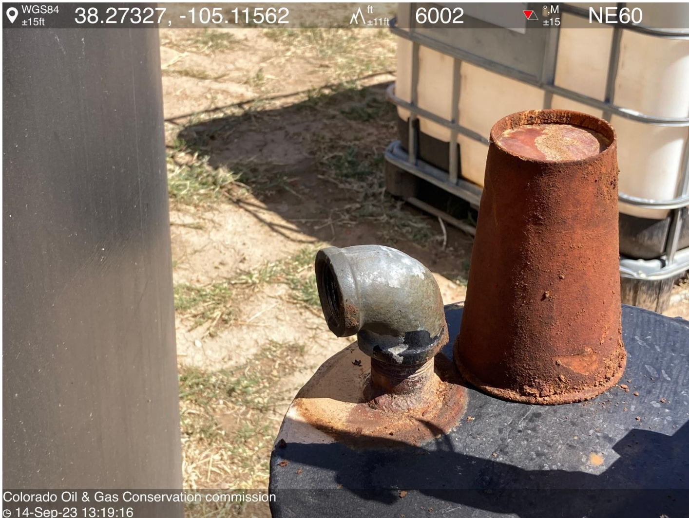
PHOTO 11: SEPARATOR IN LINE WITH 1" T-C ANNULUS SUPPLY LINE TO TANK BATTERY IS OPEN TO ATMOSPHERE. Tanks will function as sealed and ventless with gas released only through a vapor control system or properly sized pressure relief valve. per Rule 608.a.(9). 24 HOURS TO ADDRESS THIS CORRECTIVE ACTION.
