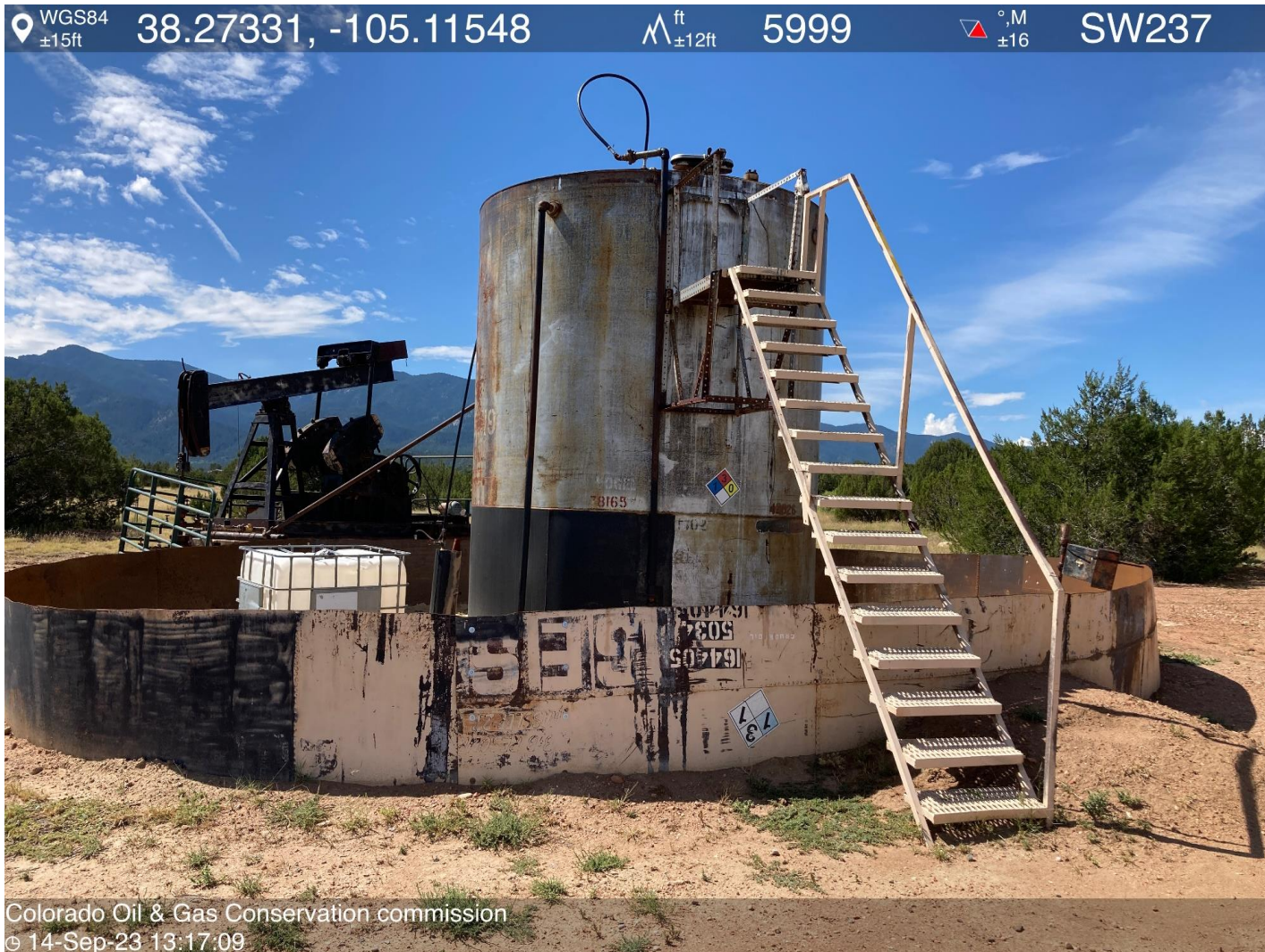
PHOTO 4: TANK BATTERY/ TANK CONTENT AND CAPACITY NOT POSTED AT TANK BATTERY. POST LABELS/SIGNS PER RULE 605. THIS IS THE 3 RD NOTICE FOR THIS CORRECTIVE ACTION, IMMEDIATE ACTION IS REQUIRED SUBMIT FIRR FORM WITH PHOTOS SHOWING TANK CONTENTS AND CAPACITY IMMEDIATELY.
