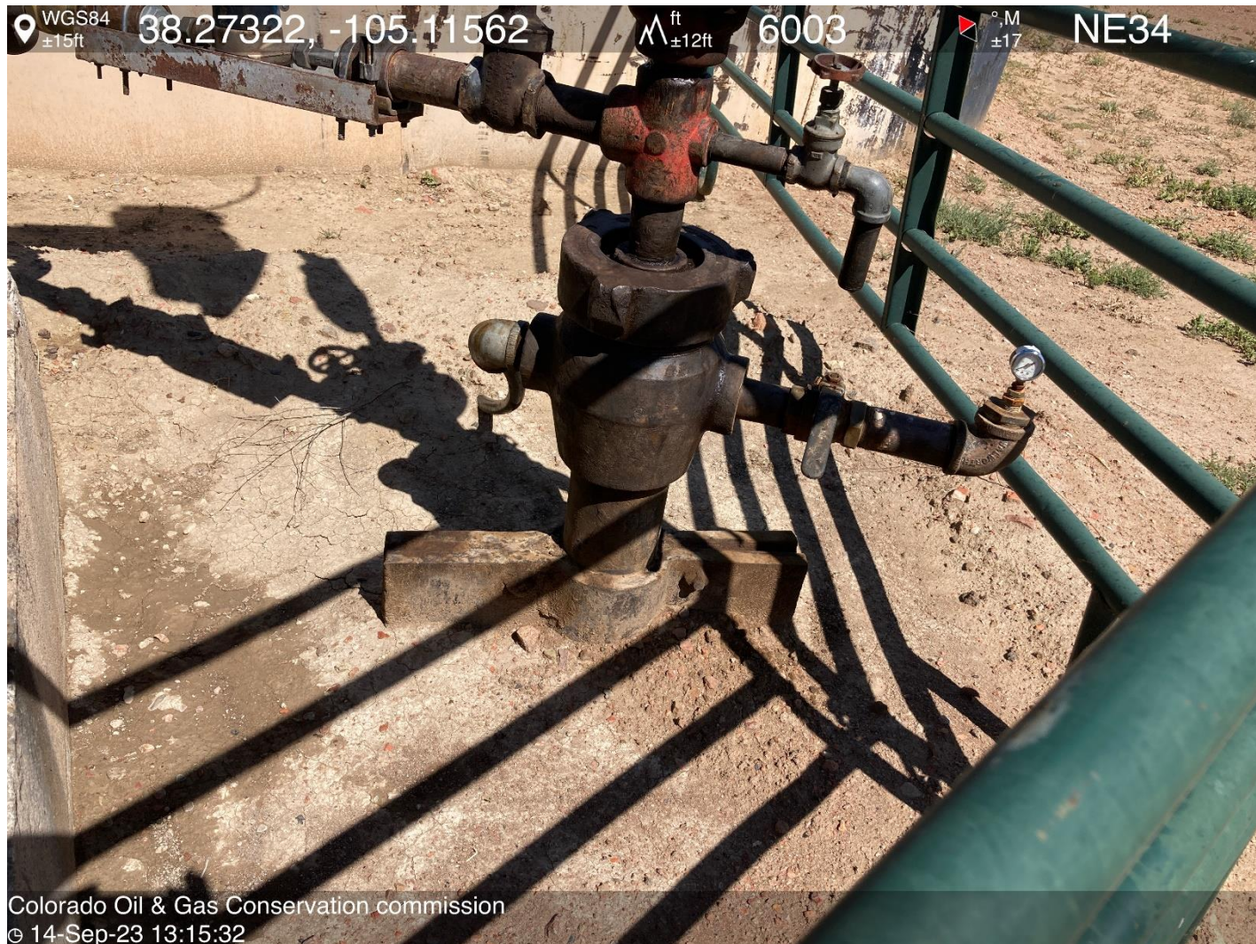
PHOTO 6: Bradenhead inaccessible or not visible (THERE DOES NOT APPEAR TO BE A BRADENHEAD INSTALLED IN WELLHEAD TREE). Install appropriate fittings to allow bradenhead visual inspection as per Rule 419.a.(1), (2). THIS IS THE 3 RD NOTICE FOR THIS CORRECTIVE ACTION, IMMEDIATE ACTION IS REQUIRED.
