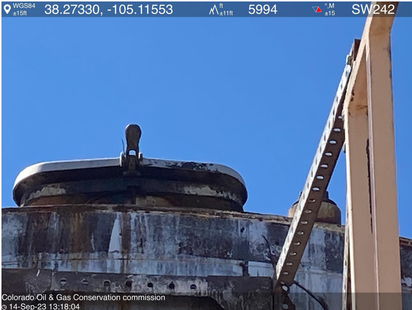
PHOTO 7: GAUGE HATCH IS NOT LATCHED. Close and seal gauge hatches when not accessing tank per Rule 608.a.(9). 24 HOURS TO ADDRESS.
