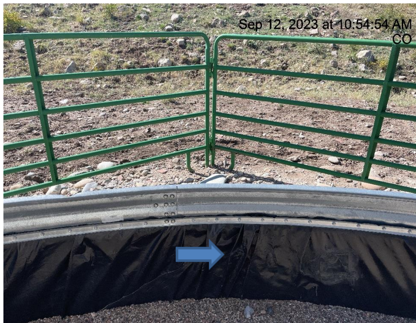
Photo # 8865 Hole in secondary containment liner/liner needs maintenance
