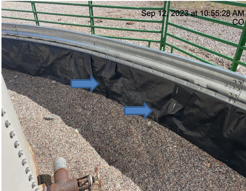
Photo # 8867 Holes in secondary containment liner/liner needs maintenance
