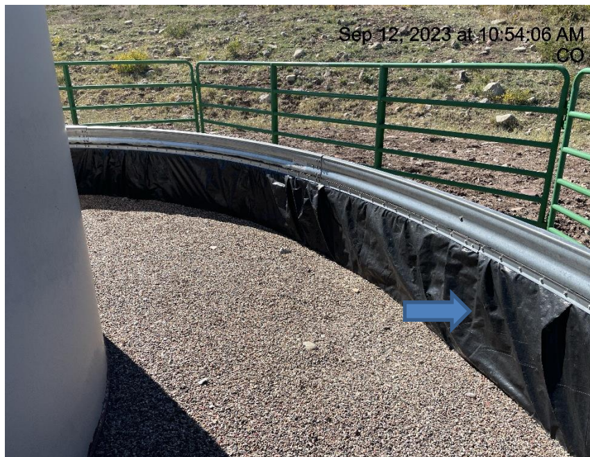
Photo # 8862 Hole in secondary containment liner/liner needs maintenance
