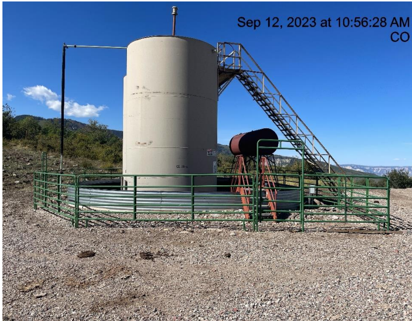
Photo # 8870 Tank battery lacks required signage
