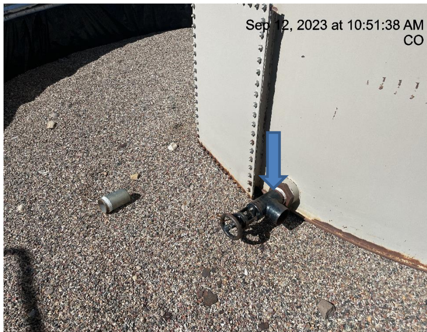
Photo # 8851 Open ended load line
