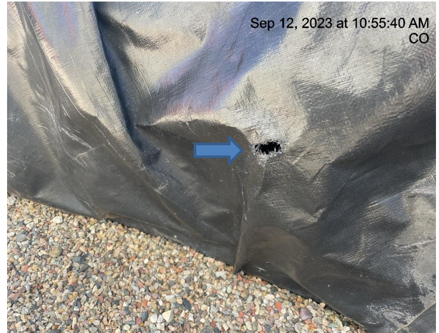
Photo # 8869 Hole in secondary containment liner/liner needs maintenance
