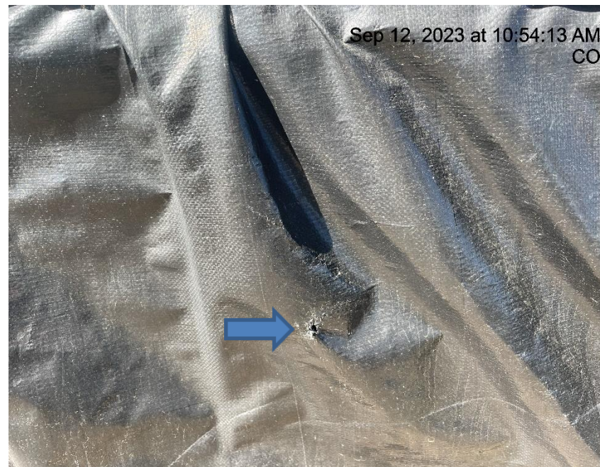
Photo # 8863 Hole in secondary containment liner/liner needs maintenance
