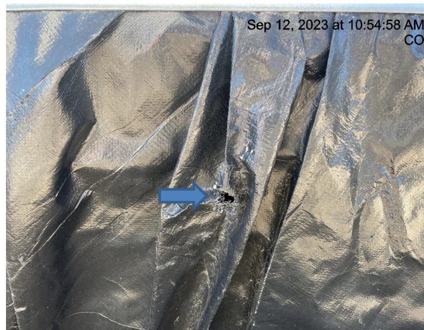
Photo # 8866 Hole in secondary containment liner/liner needs maintenance
