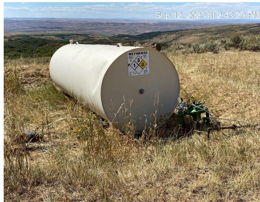
Inadequate tank berm
