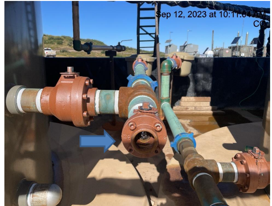
Photo # 8799 Open ended load line
