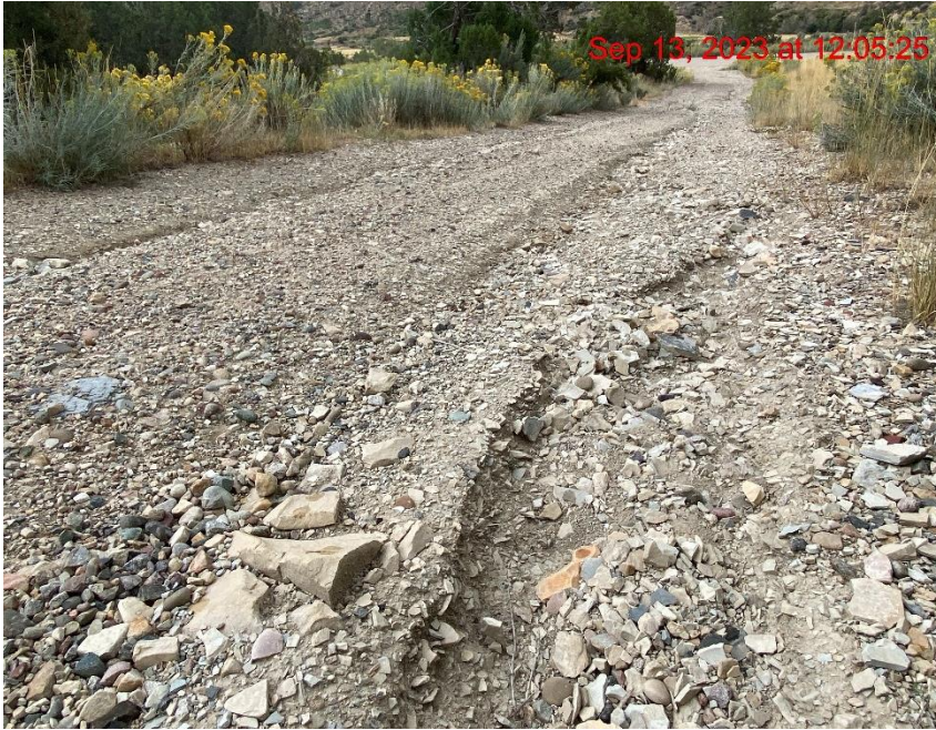
Rill Erosion Cutting Through Access Road – Photo #06380
