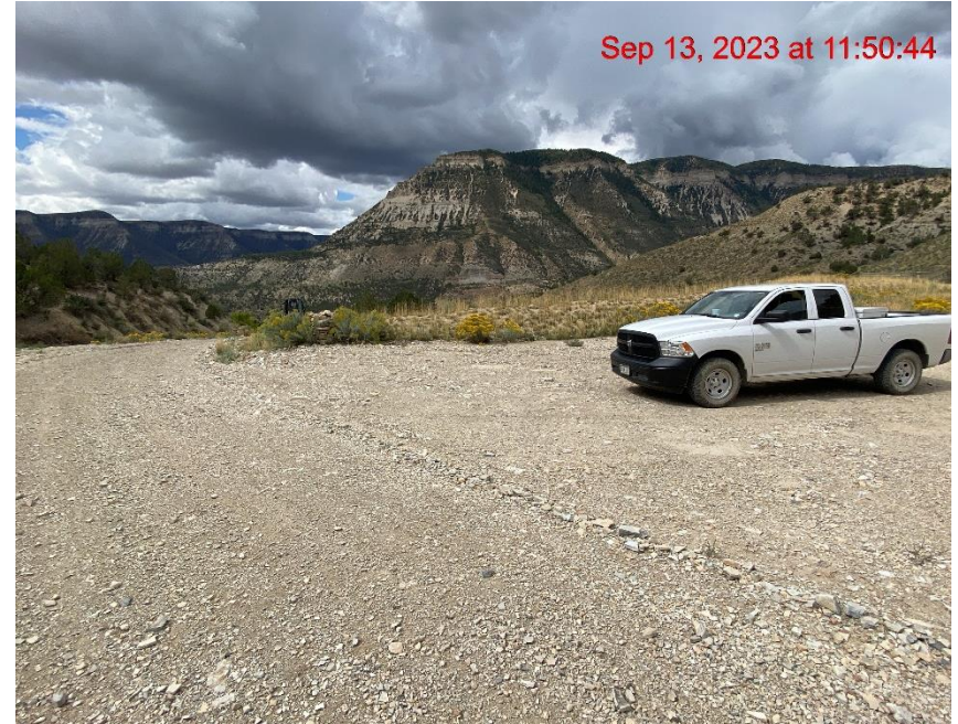
Insufficient Vehicle Tracking BMPs at Location Entrance/Exit – Photo #06374
