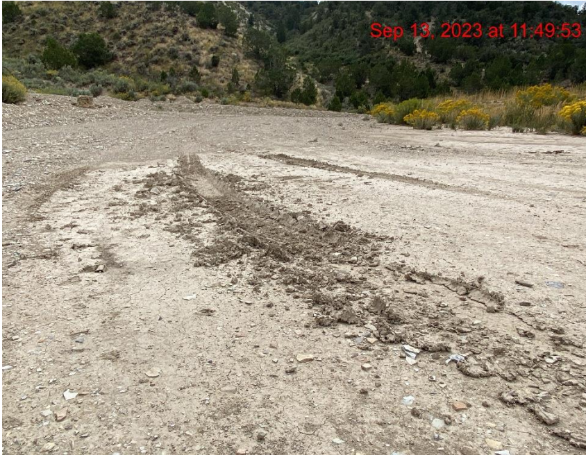
Location Lacks Stabilization – Photo #06373
