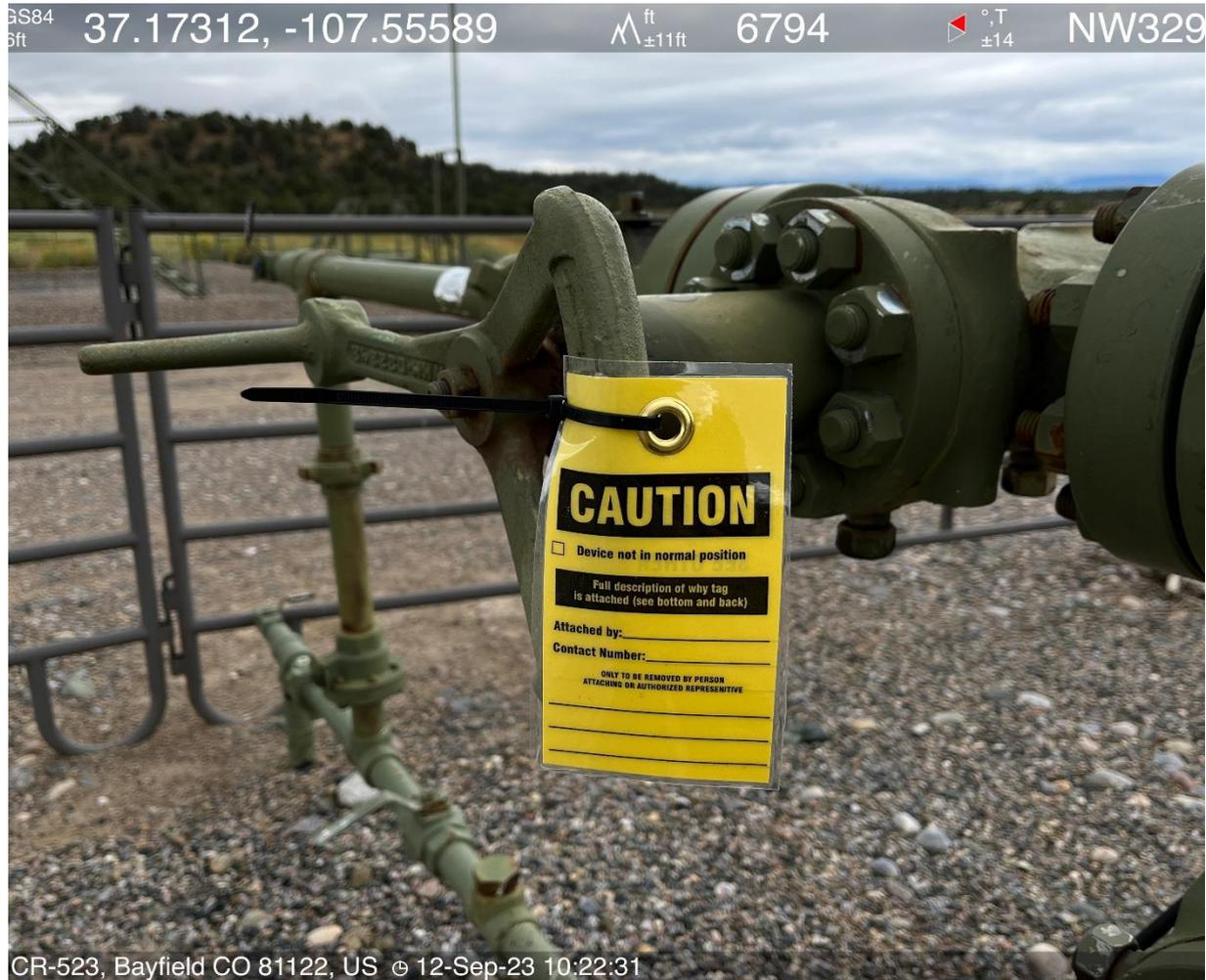
Photo #6 View of valve with audible gas leak.
