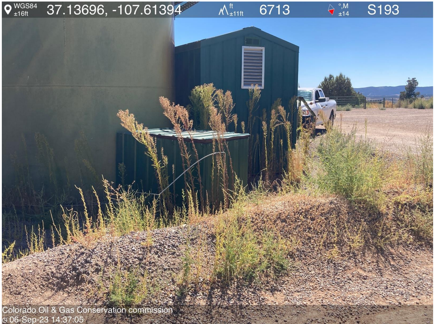
PHOTO 12: Tall weeds on and inside berms. Maintain berms/ remove weeds along with there root structures per rule 605.a. ca date 10-6-2023.
