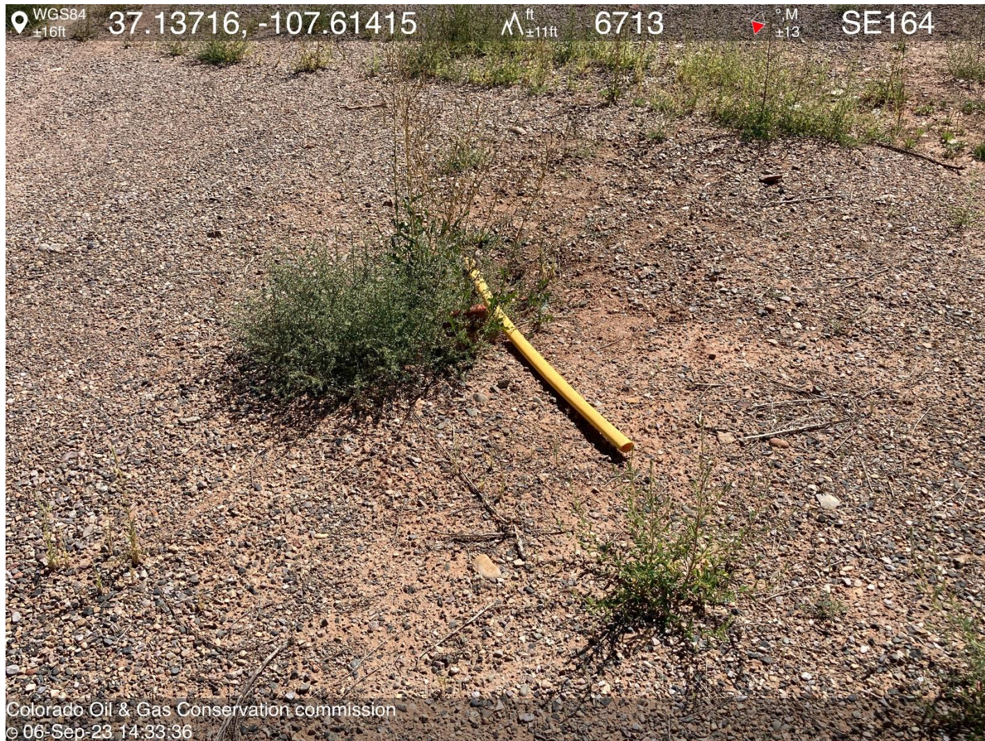
PHOTO 14: There are several anchor markers down or missing throughout location. Install proper guy line markers per Rule 1003.a ca date 10-6-2023.
