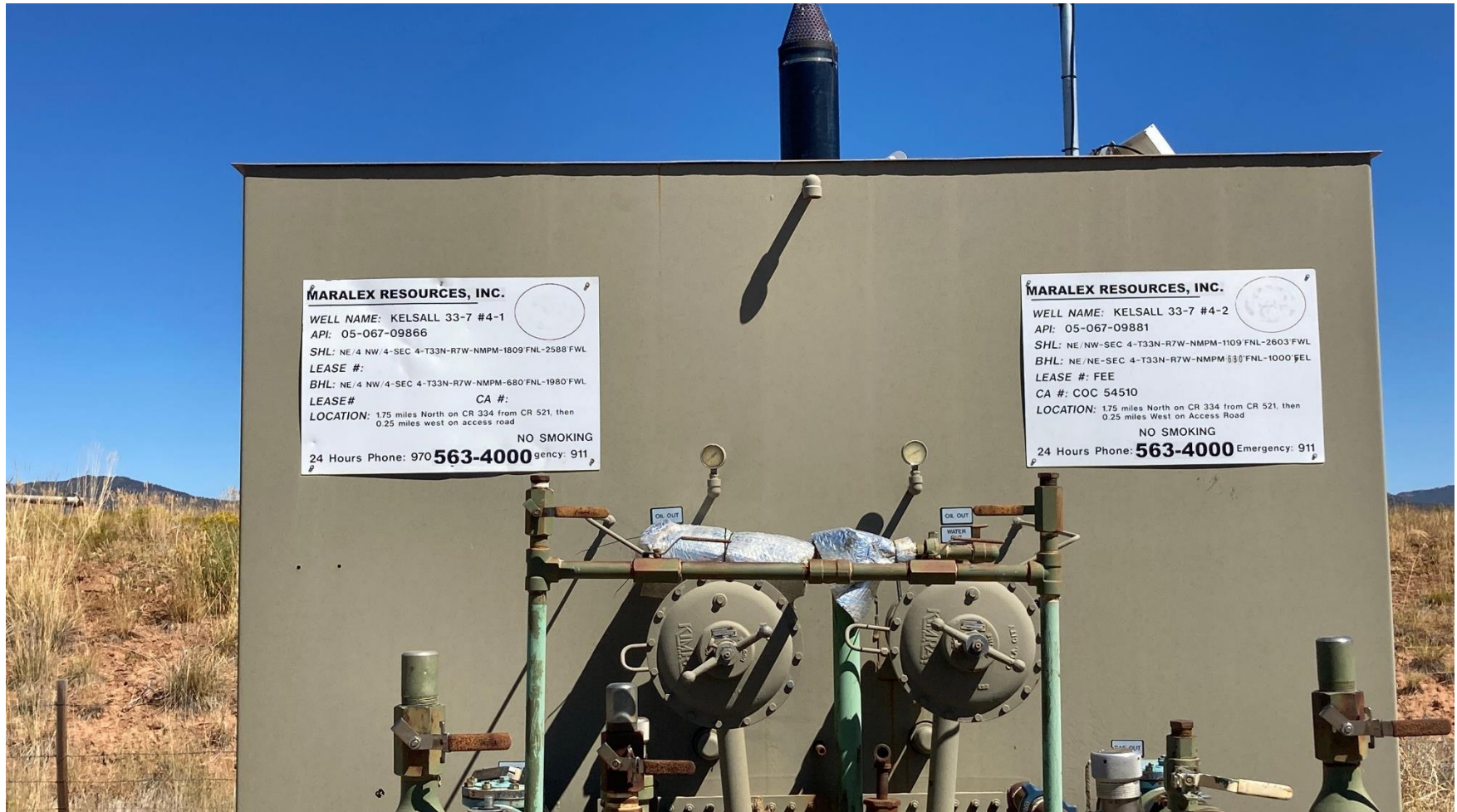
PHOTO 1: WELL SIGN/ METER AND FIRED SEPARATOR HOUSE.
