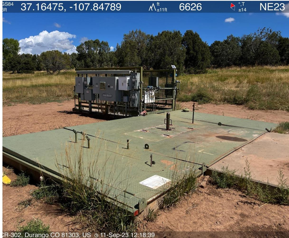
Photo #7 View of buried wellhead cellar.
