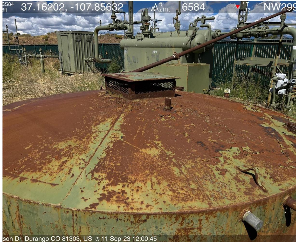
Photo #4 View of inadequate paint on produced water tank.
