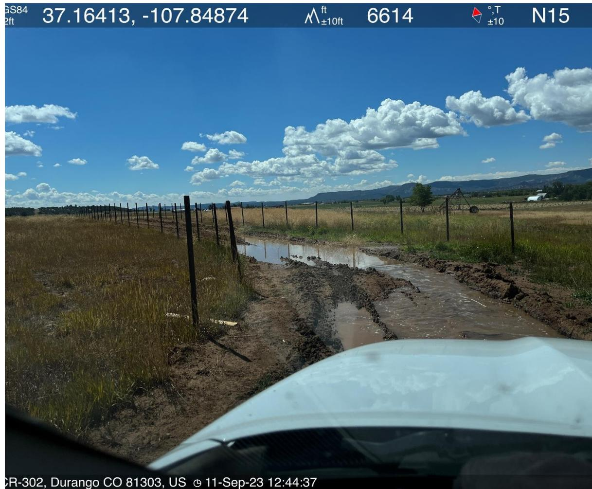
Photo #3 View of access road rutting and irrigation water.
