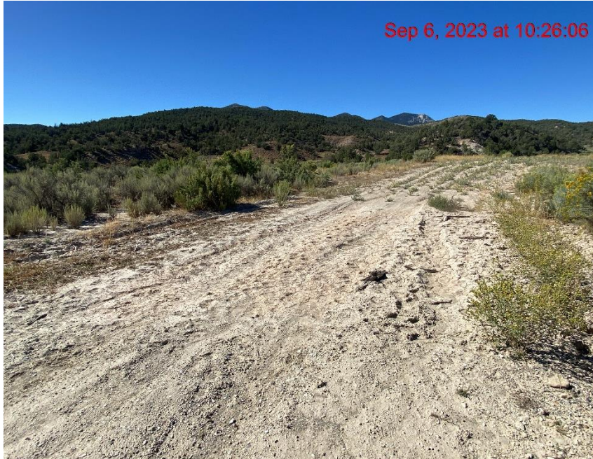
Access Road Lacks Stabilization – Photo #06285
