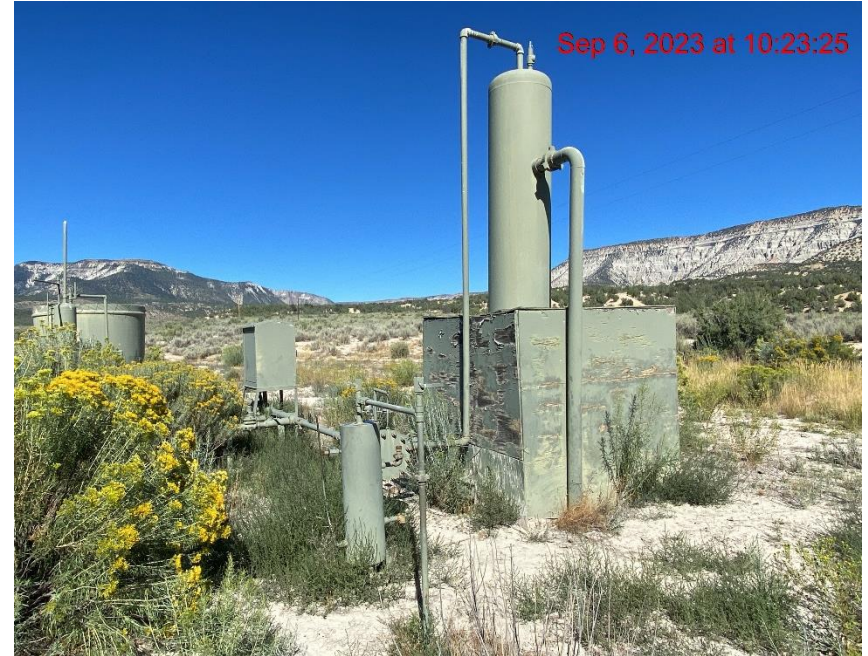
Separators/Gas Meter Run/Weeds – Photo #06279
