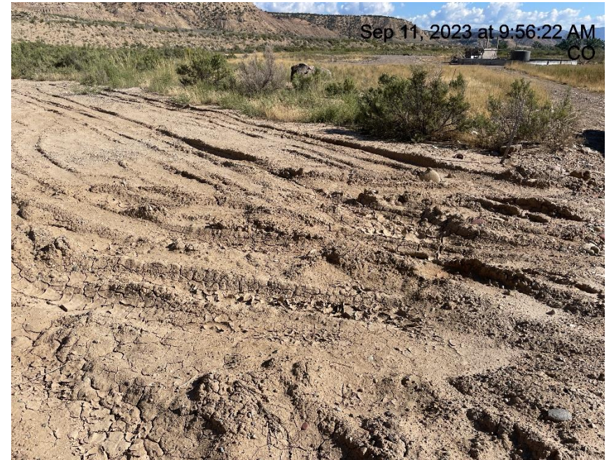
Photo # 8715 Lack of stabilization/compaction on location
