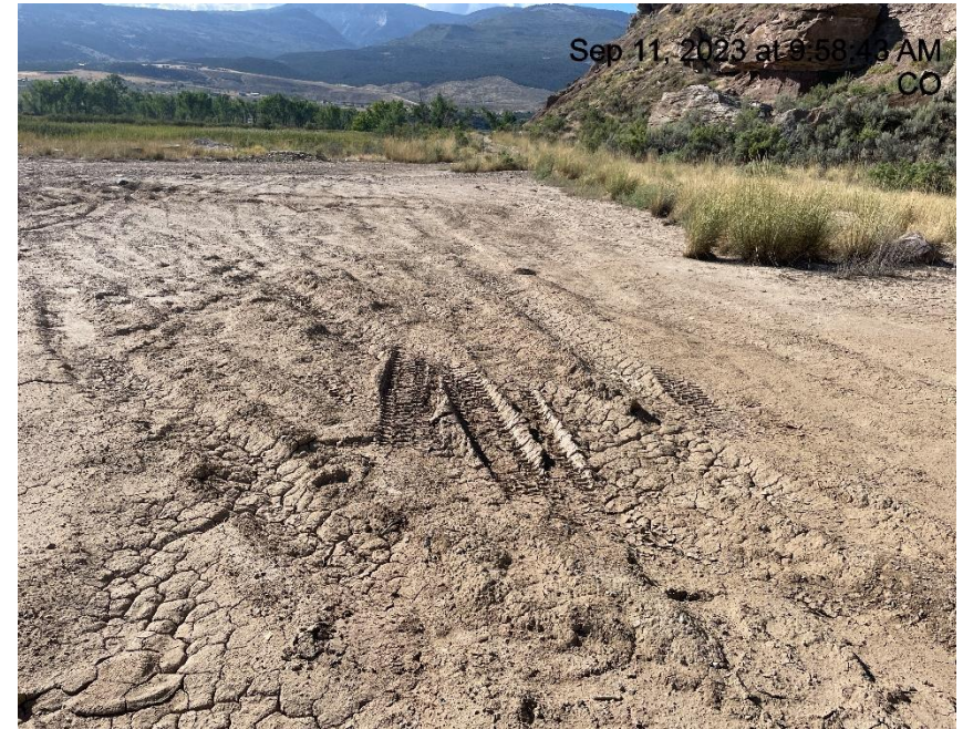
Photo # 8725 Lack of stabilization/compaction on location
