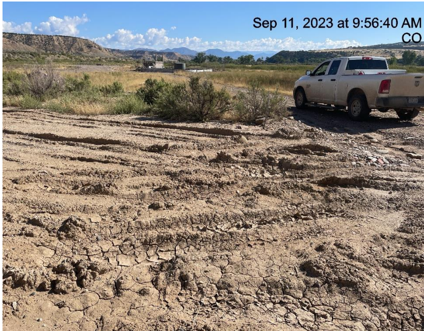
Photo # 8717 Lack of stabilization/compaction on location
