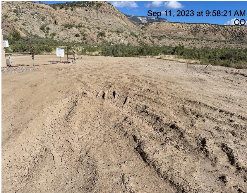
Photo # 8723 Lack of stabilization/compaction on location
