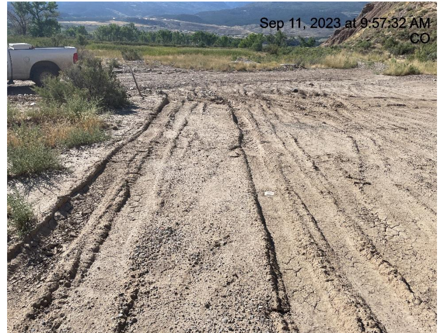
Photo # 8722 Lack of stabilization/compaction on location
