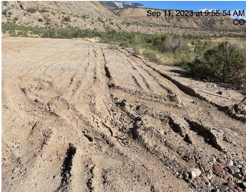
Photo # 8712 Lack of stabilization/compaction on location
