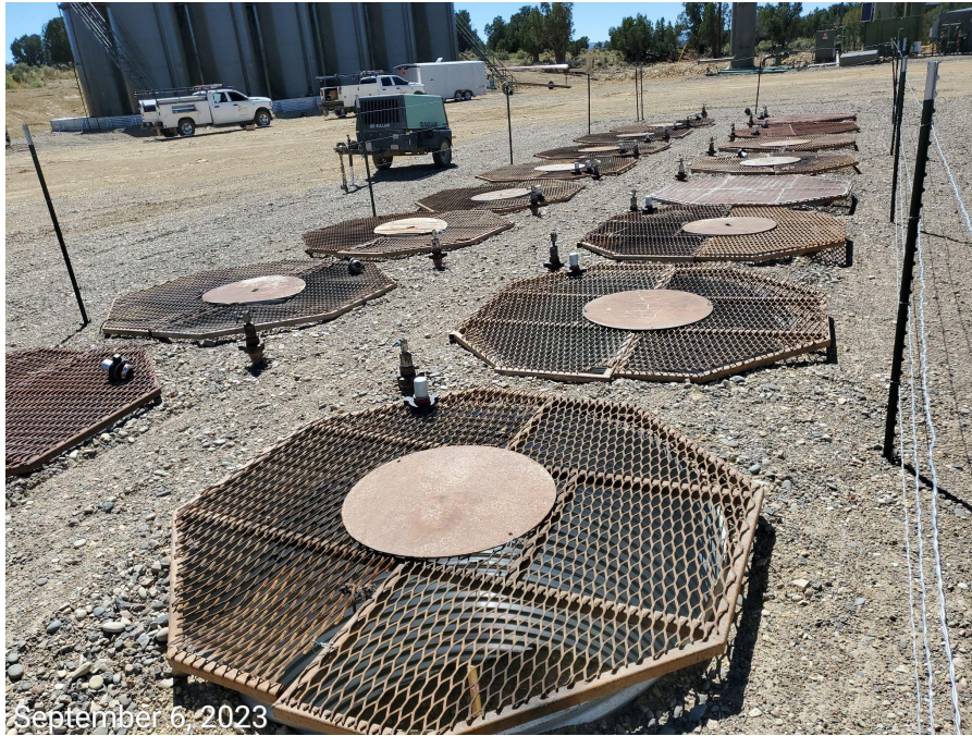
Photo 4: Cellars installed at wells, conductors not observed.
