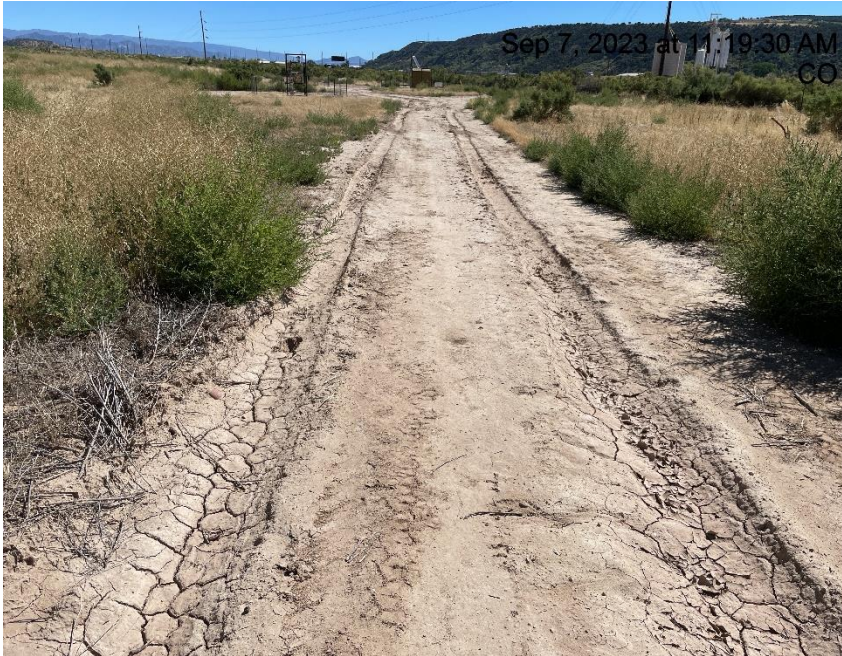
Photo # 8607 Lack of stabilization/compaction on spur road
