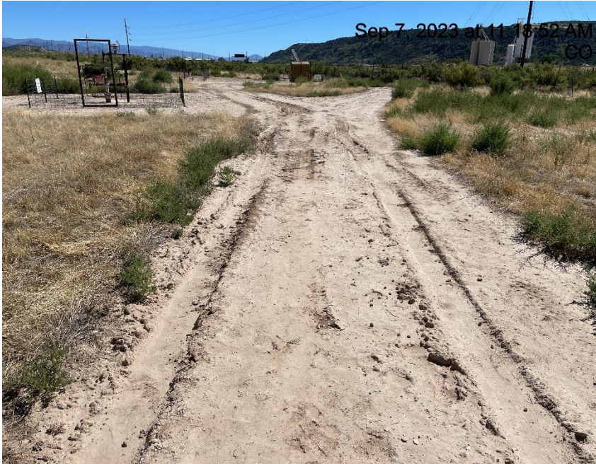
Photo # 8605 Lack of stabilization/compaction on spur road
