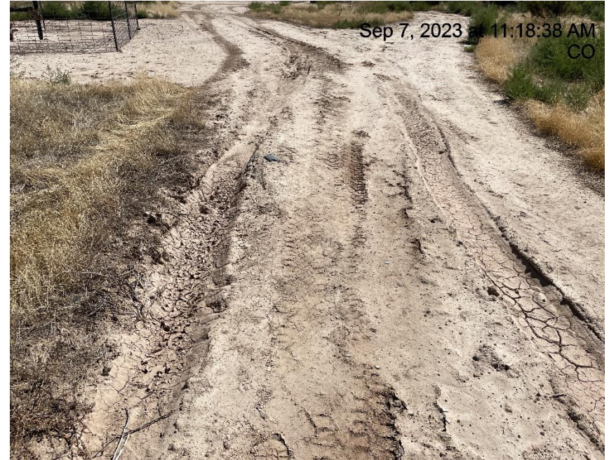
Photo # 8604 Lack of stabilization/compaction on spur road & location
