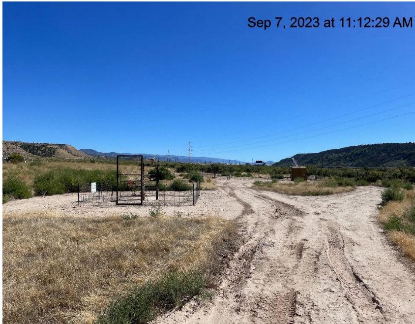
Photo # 8590 Lack of stabilization/compaction on spur road & location
