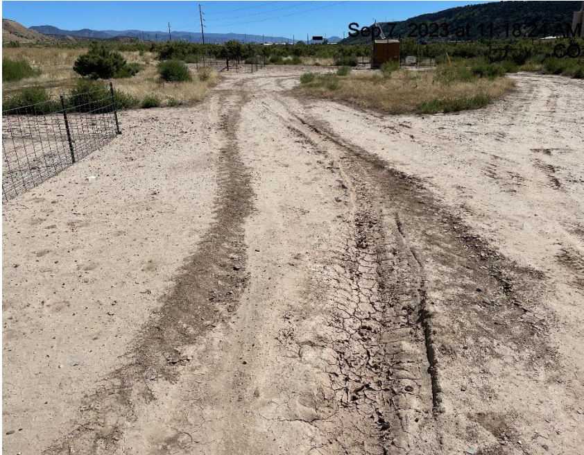
Photo # 8603 Lack of stabilization/compaction on location
