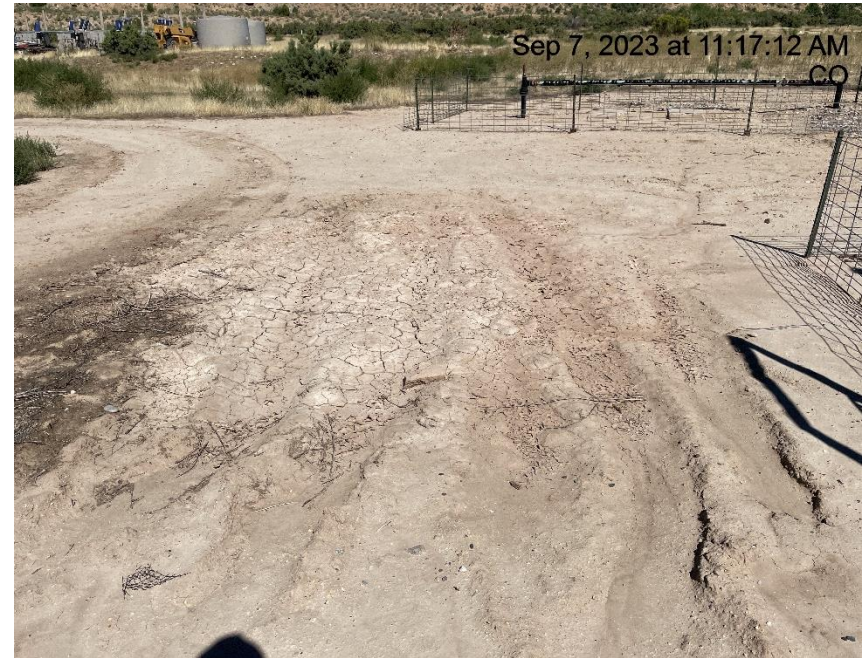
Photo # 8599 Lack of stabilization/compaction on location
