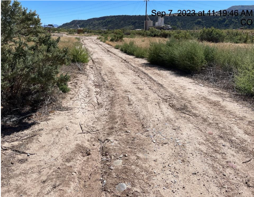
Photo # 8609 Lack of stabilization/compaction on spur road
