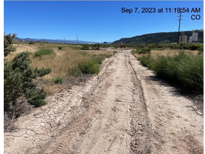
Photo # 8610 Lack of stabilization/compaction on spur road
