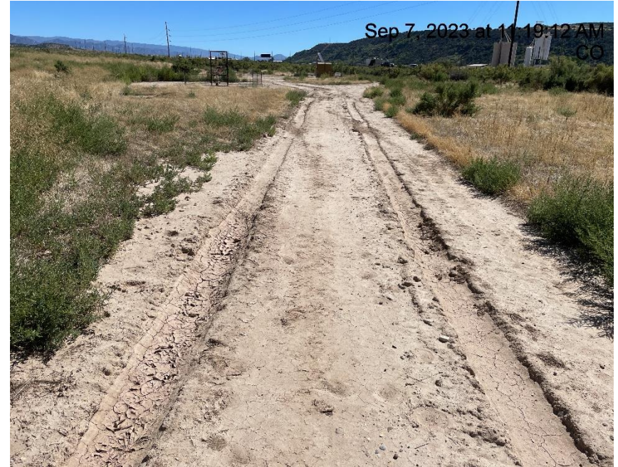
Photo # 8606 Lack of stabilization/compaction on spur road
