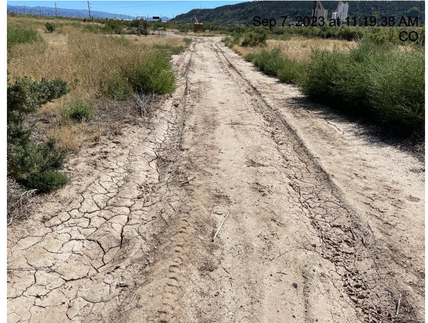
Photo # 8608 Lack of stabilization/compaction on spur road
