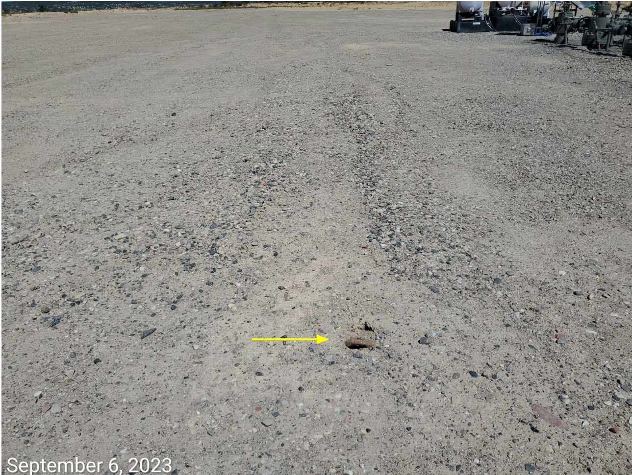
Photo 11: Photo example showing unmarked anchors on the Location.
