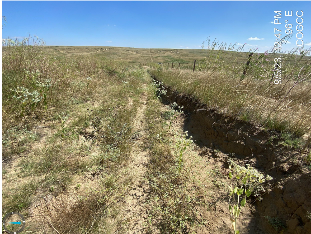
Photo 4. The former access road requires additional contouring and grading; cut banks illustrated.
