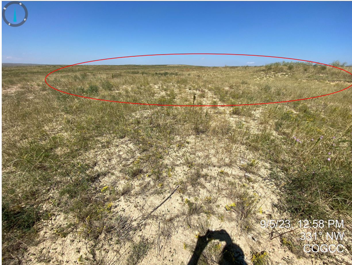
Photo 11. Taken from the center portion of the location. Photo illustrates additional recontouring activities that are required around the former wellhead location.
