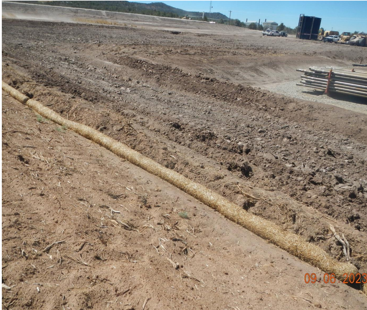
Photo #17 View of no wattle staking.
