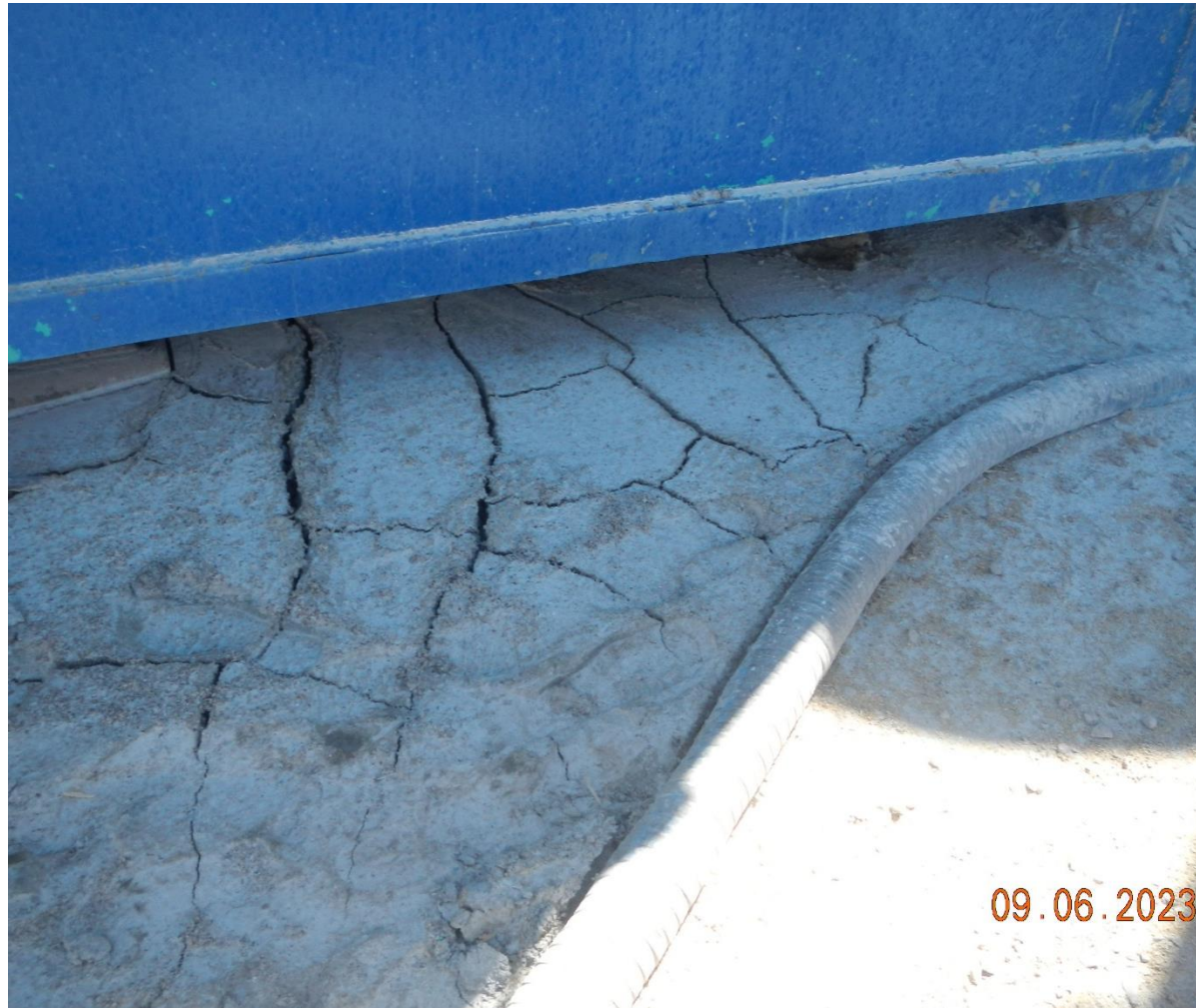
Photo #20 View of dried drilling additives.
