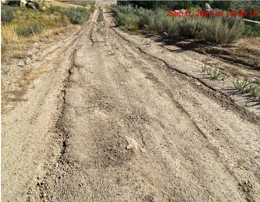
Insufficient Erosion Control/Rill Erosion on Access Road – Photo #06250
