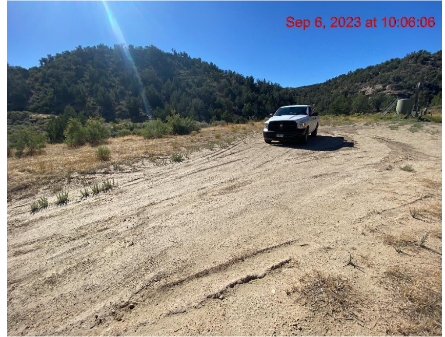
Insufficient Vehicle Tracking BMPs at Location Entrance/Exit – Photo #06249
