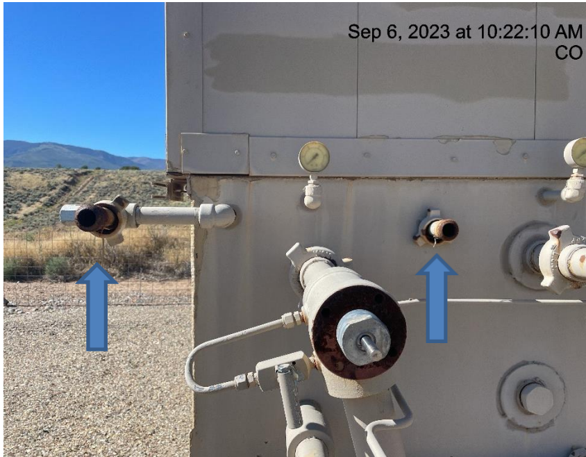
Photo # 8283 Open ended piping on production unit/wildlife hazard
