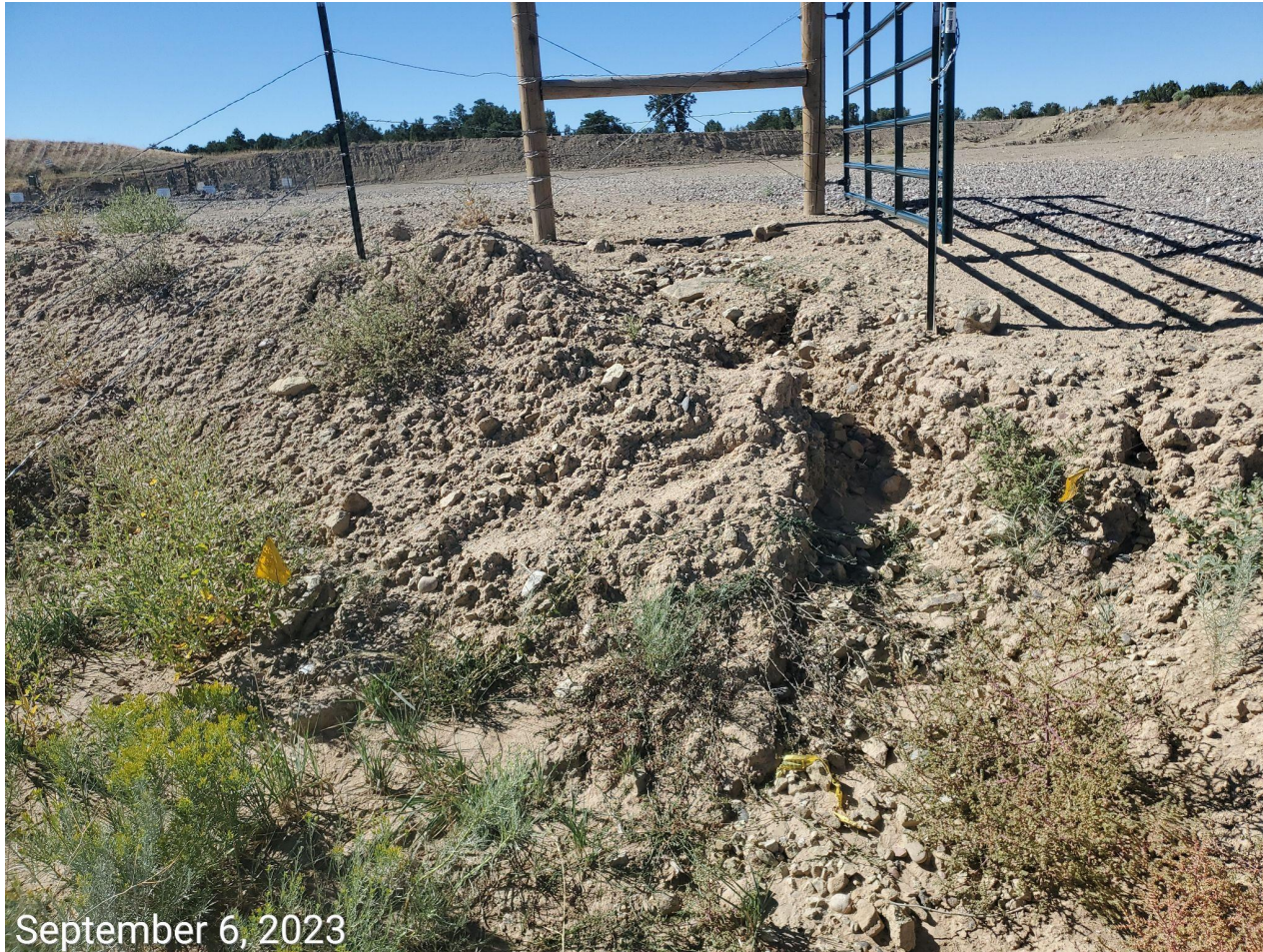
Photo 3: Photo example of erosion degradation at the northern location entrance; erosion apparent on both the east and west sides of the location entrance road.
