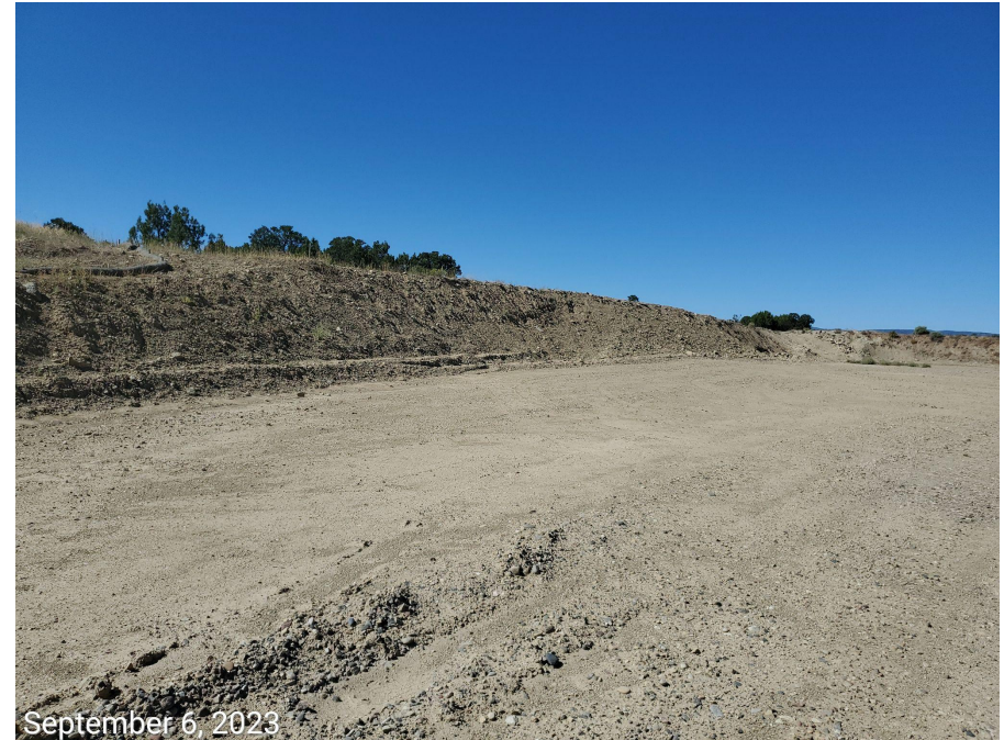
Photo 11: Cut slopes lack stabilization and BMPs to minimize erosion and degradation.
