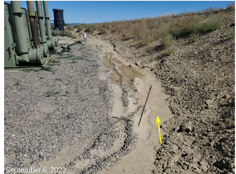
Photo 11: Cut slopes lack stabilization and BMPs to minimize erosion and degradation. Arrow shows sediment deposition due to erosion at the cut slopes.
