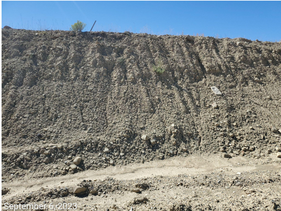
Photo 11: Cut slopes lack stabilization and BMPs to minimize erosion and degradation.
