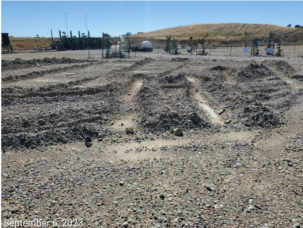
Photo 10: Photos show unstabilize soils remain on the working pad surface.
