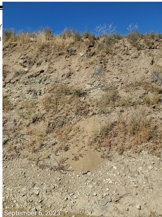
Photo 12: Cut slopes lack stabilization and BMPs to minimize erosion and degradation.
