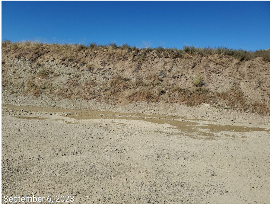
Photo 12: Cut slopes lack stabilization and BMPs to minimize erosion and degradation.
