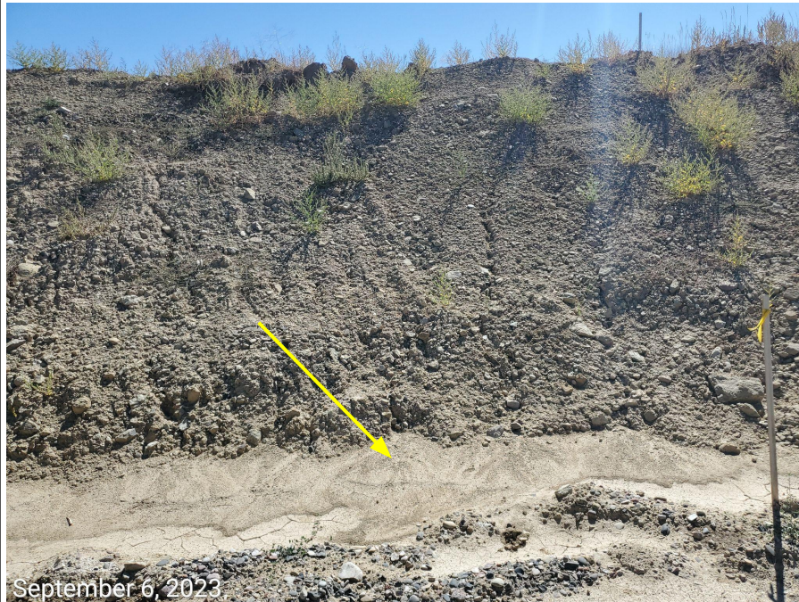
Photo 11: Cut slopes lack stabilization and BMPs to minimize erosion and degradation. Arrow shows sediment deposition due to erosion at the cut slopes.
