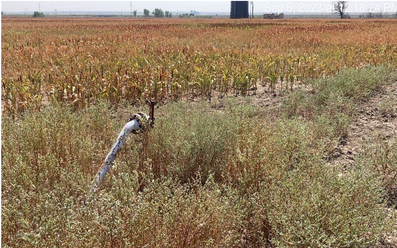
Photo 1. Facing southeast at the abandoned wellsite. There is an abandoned pipe riser that still remains and must be removed. Pipe riser is interfering with crop production.
