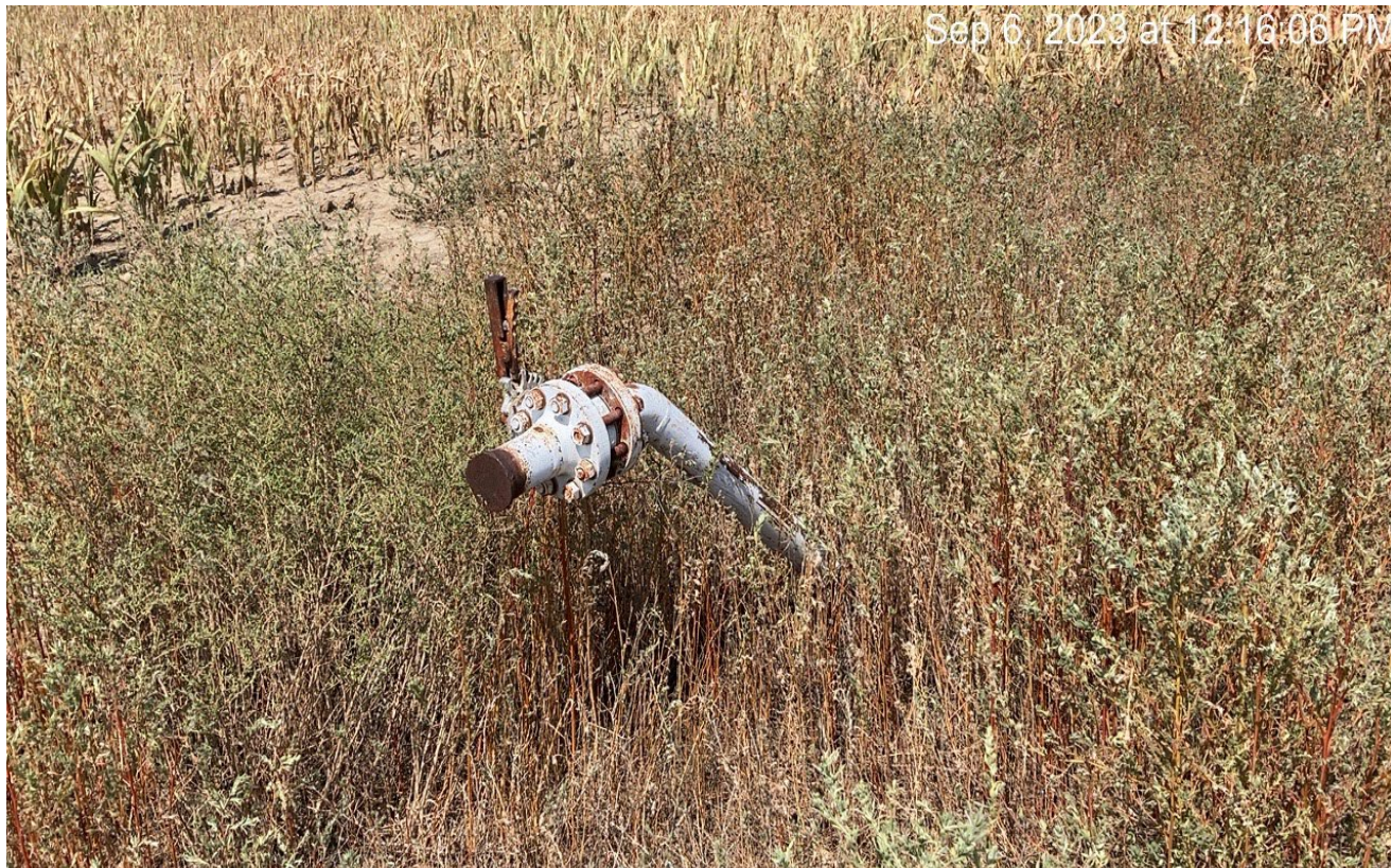
Photo 2. Abandoned capped pipe riser needs to be removed.
