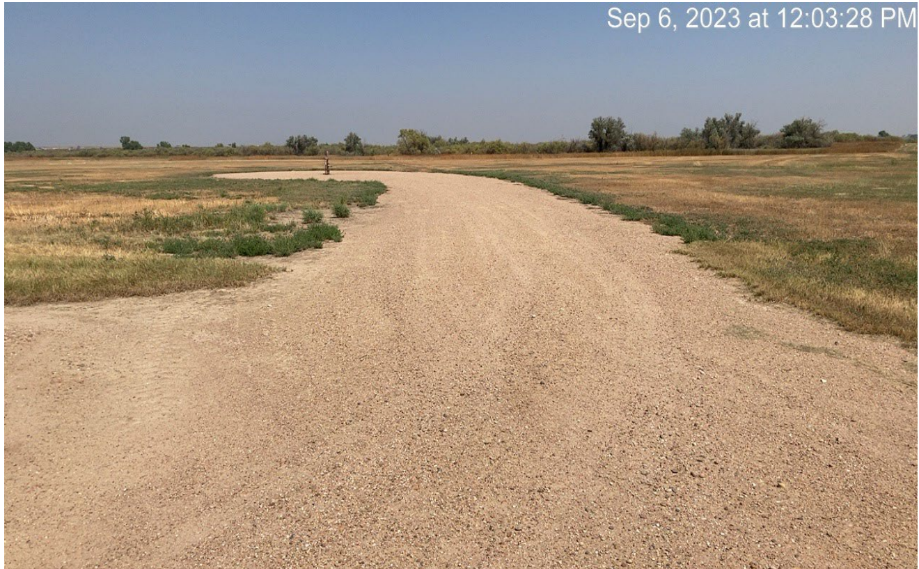
Photo 4. There is well sign posted at the wellhead. The well is a distance away from the tank battery and an addition sign should be posted at the tank battery.
