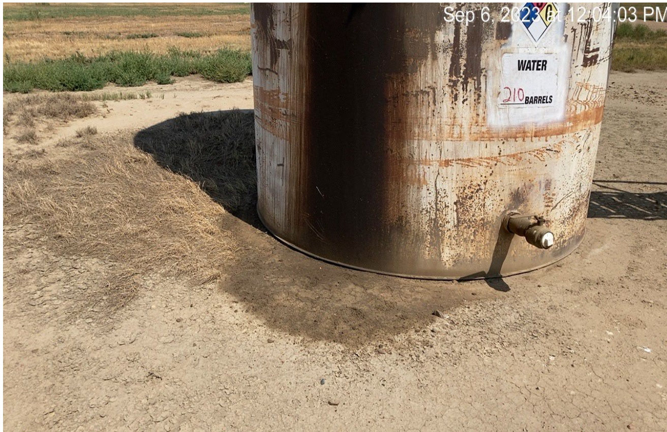
Photo 3. Facing toward the tank battery. There is oil stained soil at the pipe outlet and at the base of the tanks. Previous corrective action was not completed.
