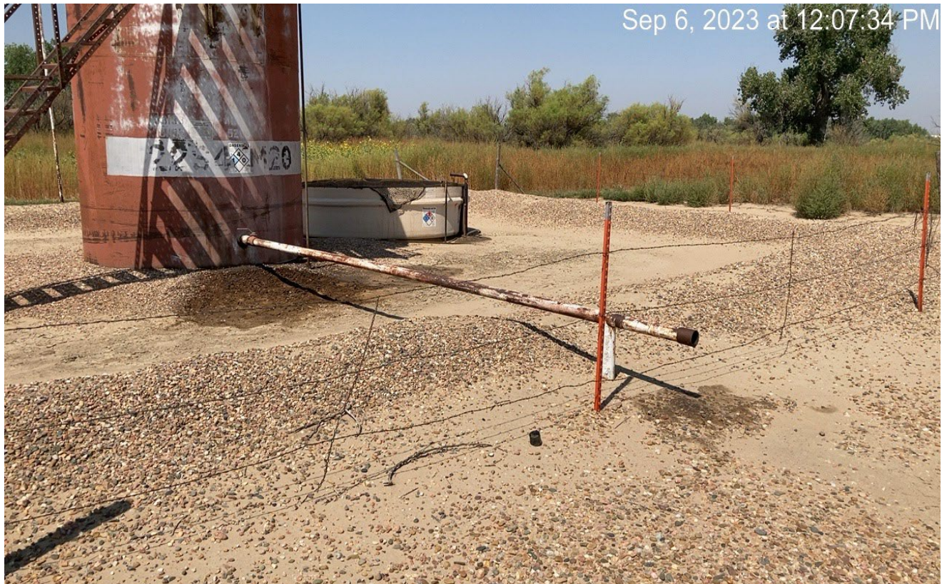
Photo 3. Facing toward the tank battery. There is oil stained soil at the pipe outlet and at the base of the tanks.
