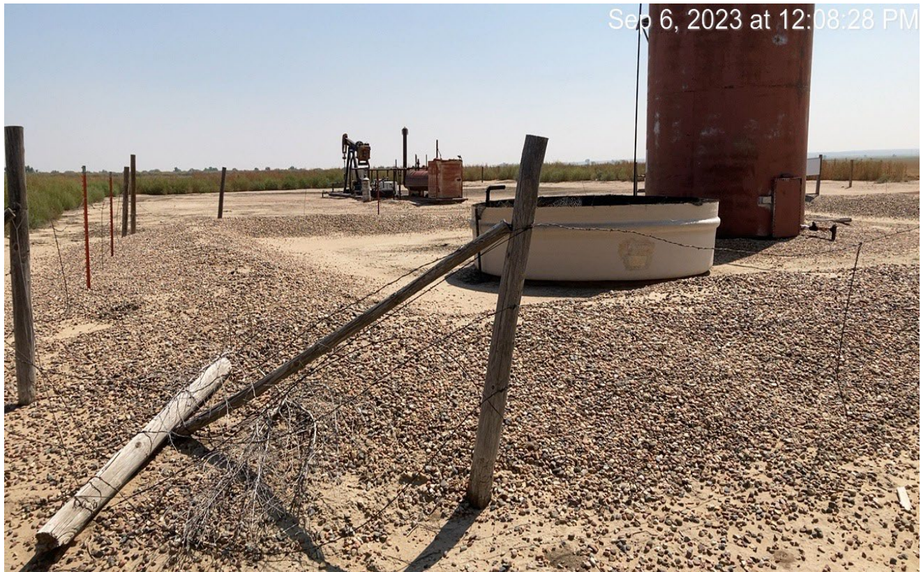
Photo 7. The fence at the northwest corner of the tank battery is in disrepair..
