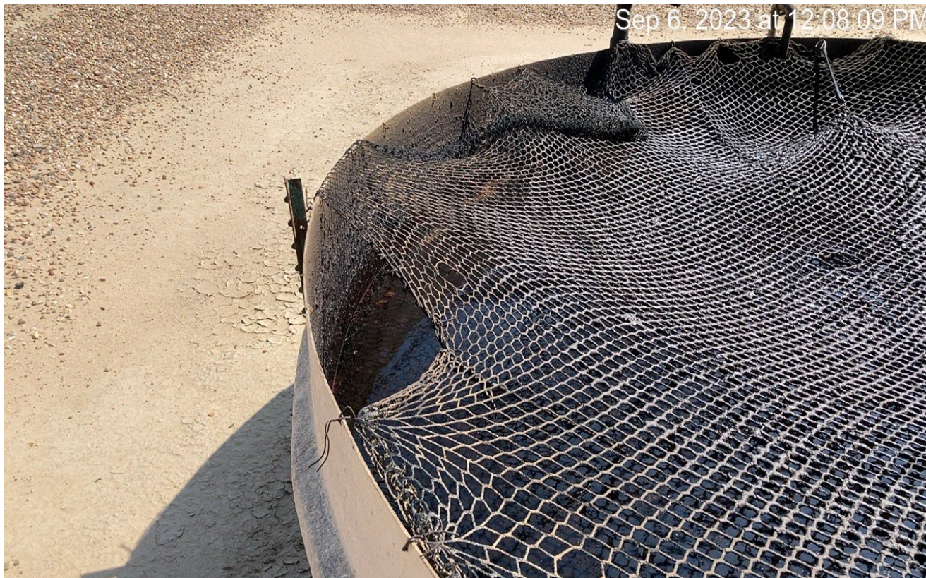
Photo 6. The netting on the open top tank is still insufficient to prevent wildlife entry. Previous corrective action was not completed.
