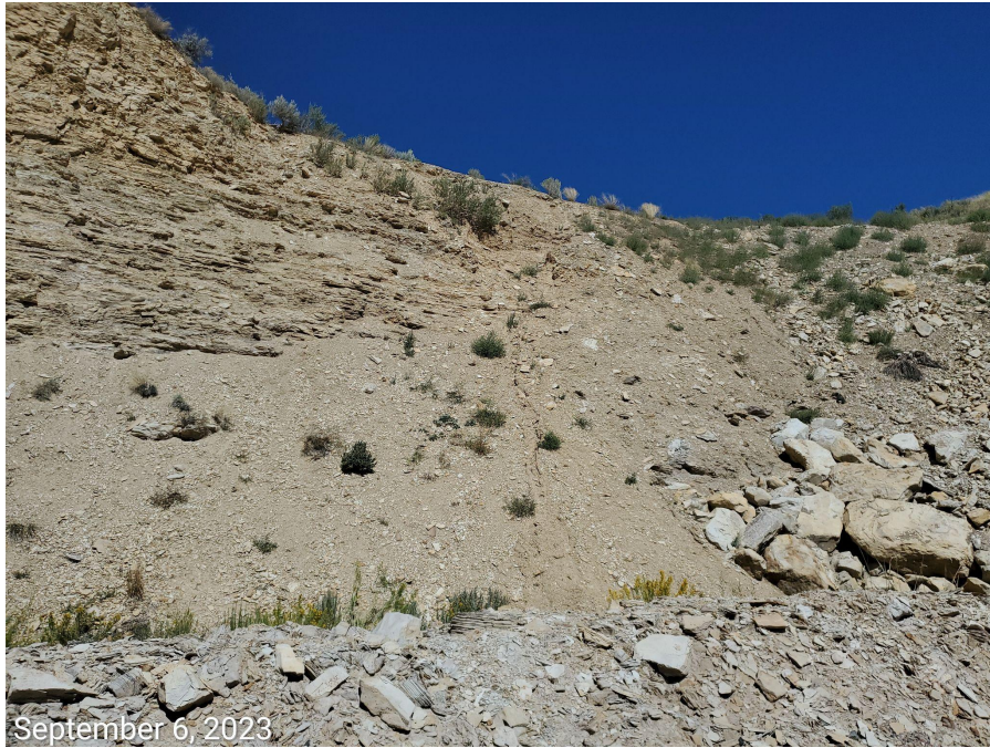
Photo 6: Photos taken from the northeastern cut slopes of the Location. Slopes lack stabilization.
