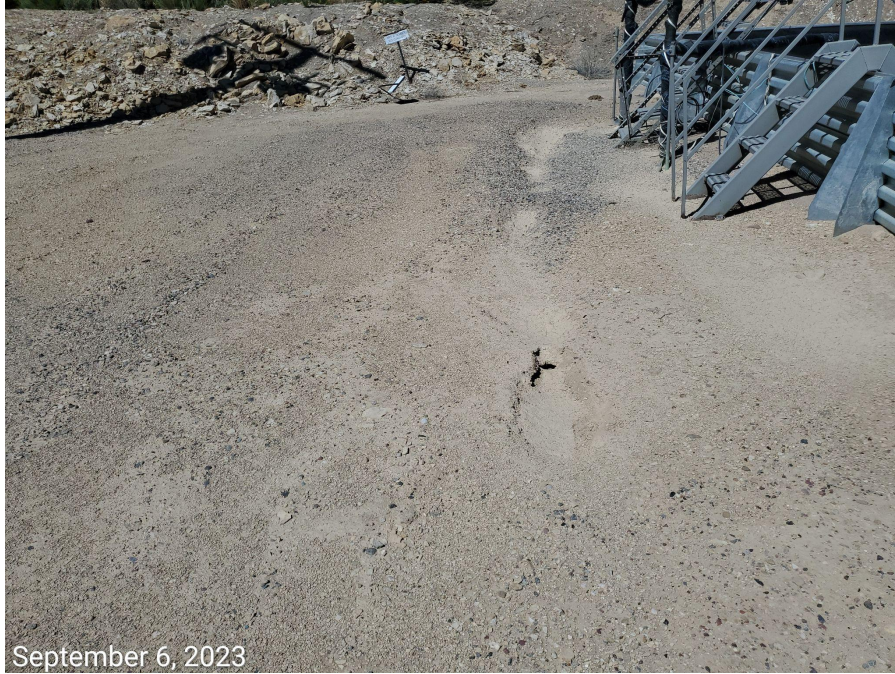
Photo 11: Subsidence concerns observed on the west end of the battery facility.
