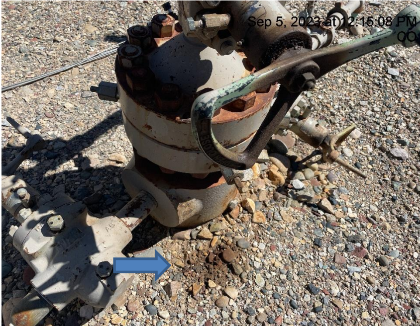
Photo # 8230 Stained soils & gravel near wellheads
