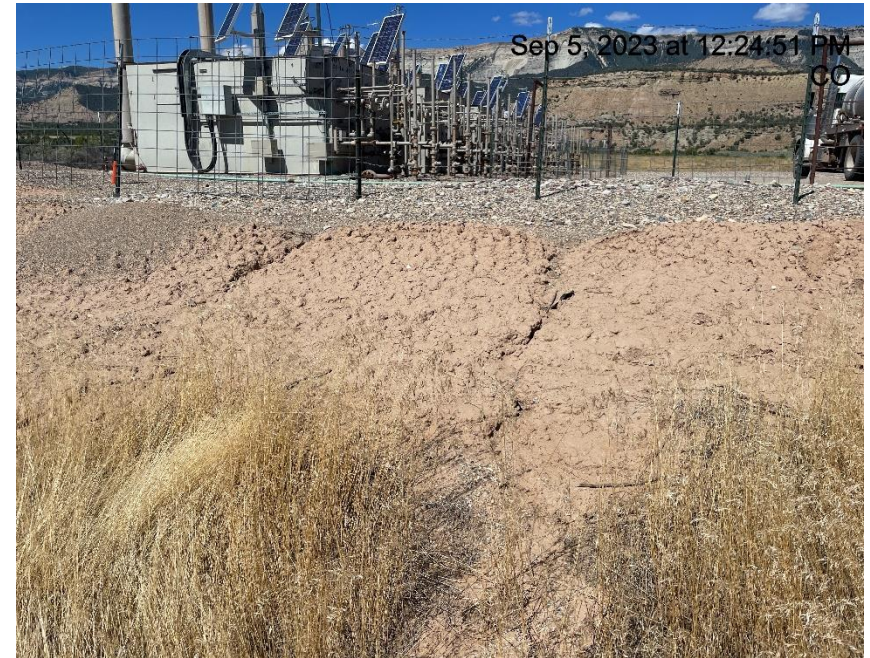
Photo # 8254 Erosion & transport of sediment off location & into a vegetated area
