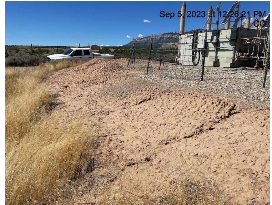
Photo # 8261 Erosion & transport of sediment off location & into a vegetated area
