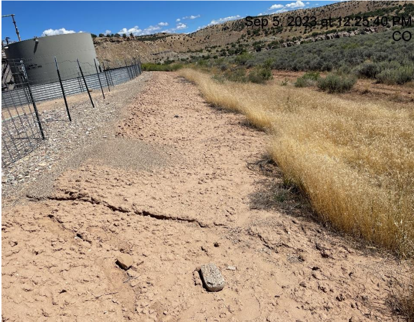
Photo # 8259 Erosion & transport of sediment off location & into a vegetated area
