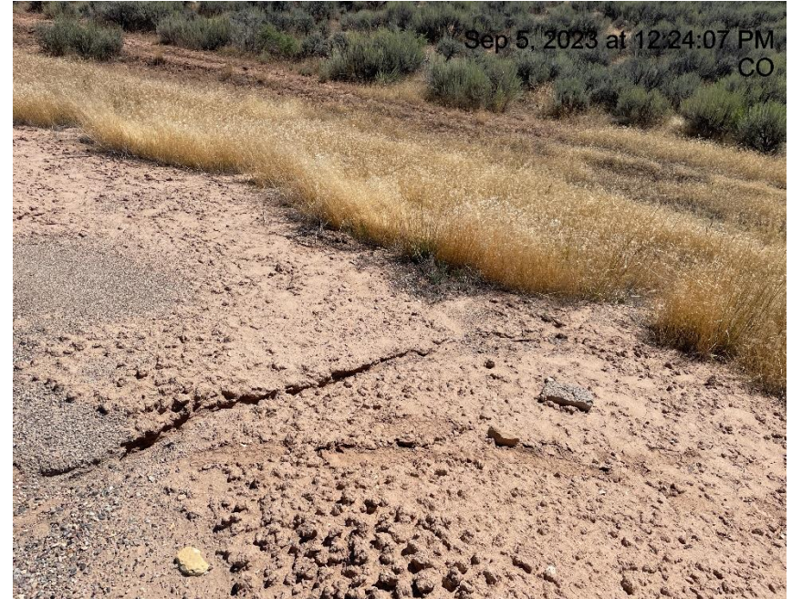
Photo # 8249 Erosion & transport of sediment off location & into a vegetated area
