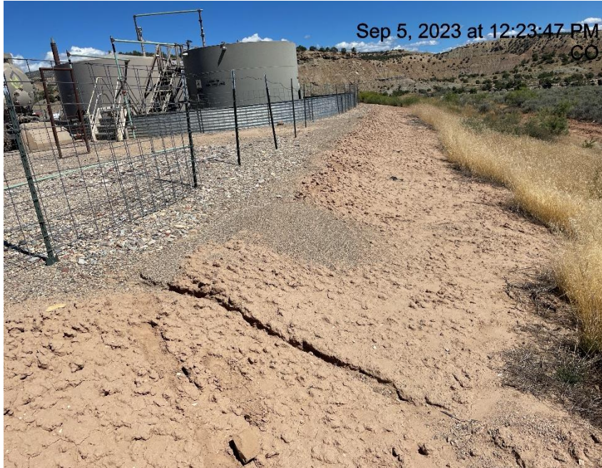
Photo # 8248 Erosion & transport of sediment off location & into a vegetated area
