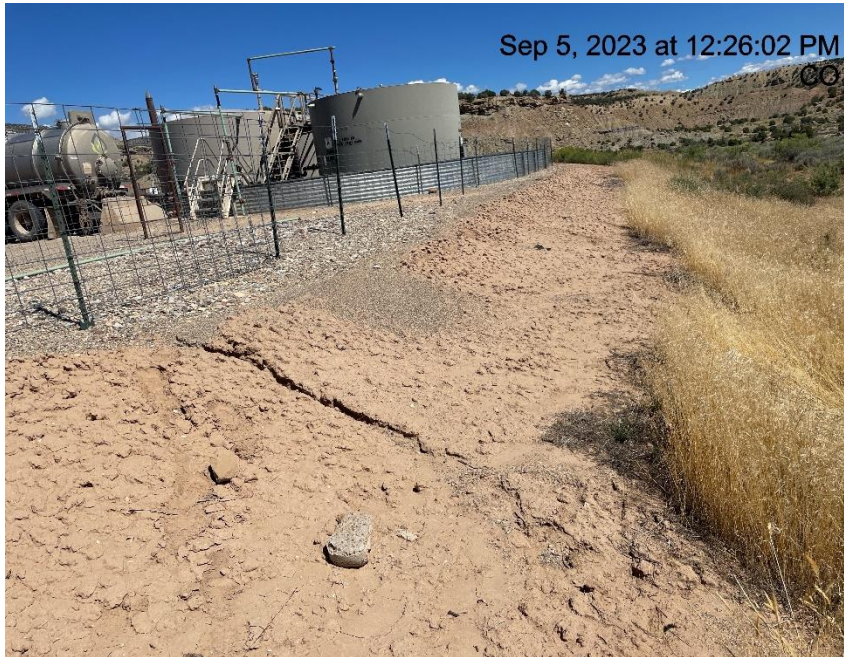
Photo # 8260 Erosion & transport of sediment off location & into a vegetated area
