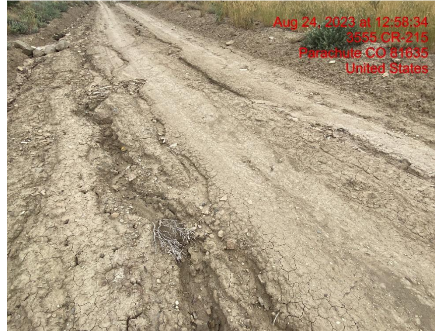
Insufficient Erosion Controls/Rill Erosion on Access Road – Photo #06192
