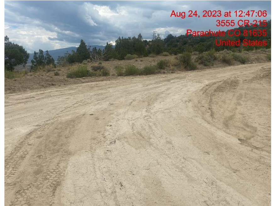
Insufficient Vehicle Tracking BMPs at Location Entrance/Exit – Photo #06190
