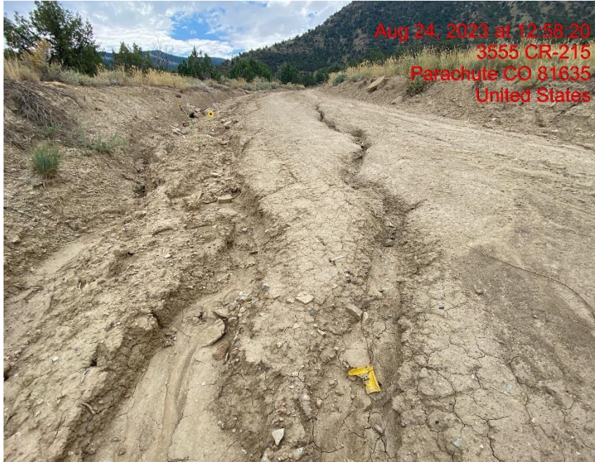
Insufficient Erosion Controls/Rill Erosion on Access Road – Photo #06191
