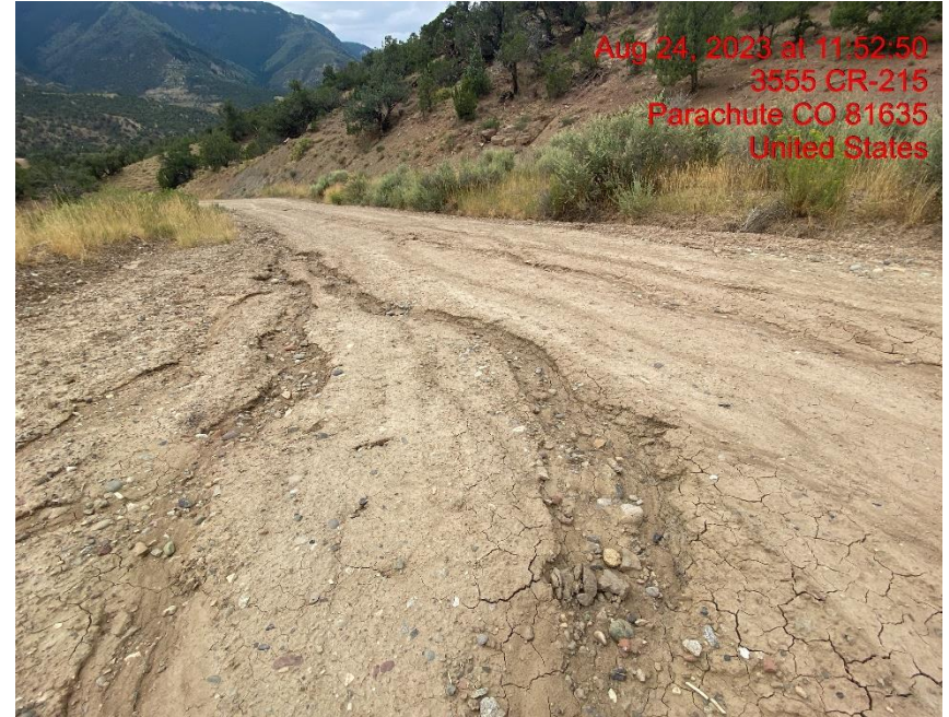
Insufficient Erosion Control/Rill Erosion on Access Road – Photo #06154
