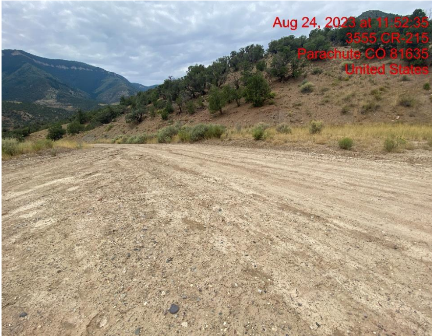
Insufficient Vehicle Tracking BMPs at Location Entrance/Exit – Photo #06153
