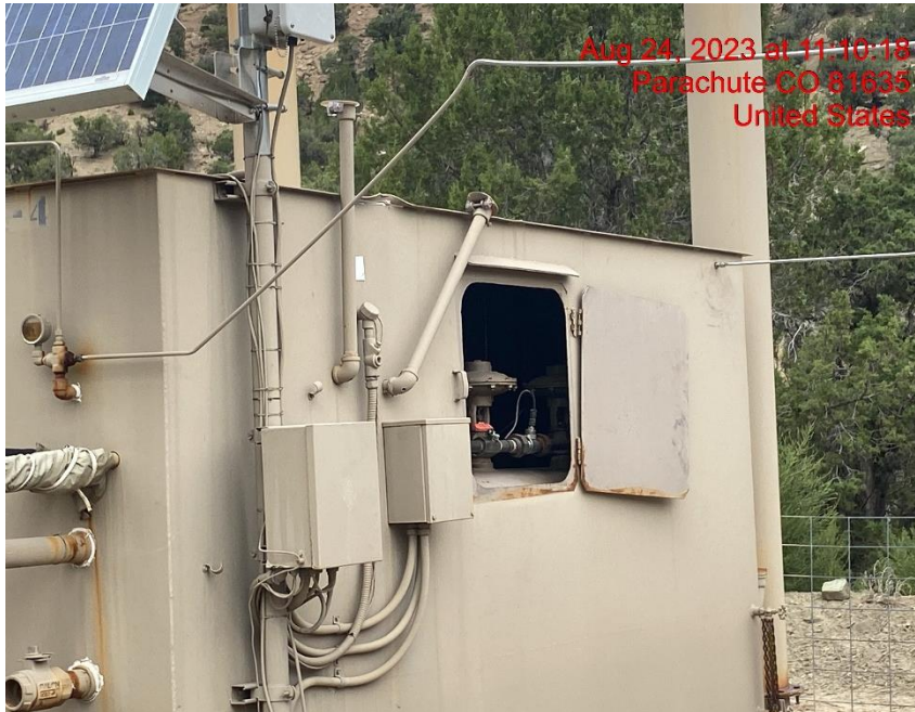
Unsecured Separator Hatches – Photo #06128
