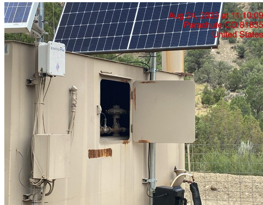
Unsecured Separator Hatches – Photo #06127
