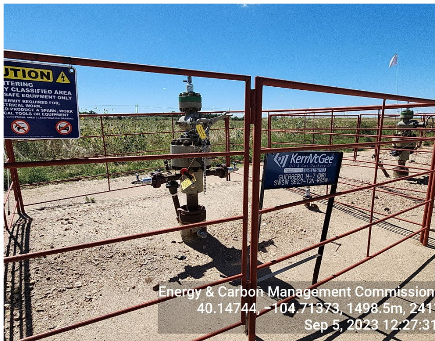
Photo 1: TA Wellhead
