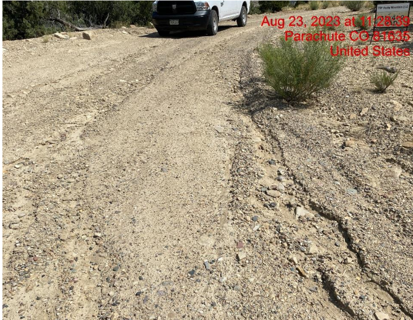
Rill Erosion on Access Road – Photo #06100
