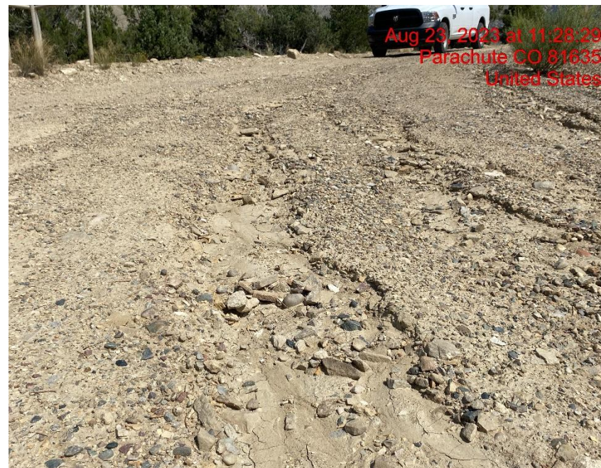
Rill Erosion on Access Road – Photo #06099
