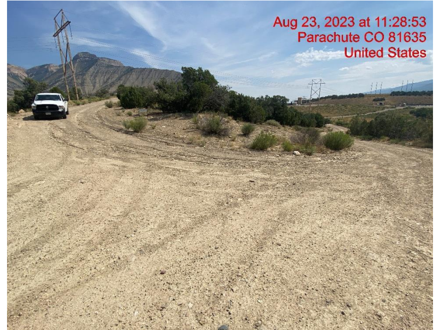
Insufficient Vehicle Tracking BMPs at Location Entrance/Exit – Photo #06101
