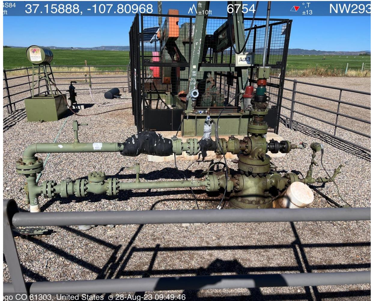
Photo #3 View of the #3 wellhead assembly.
