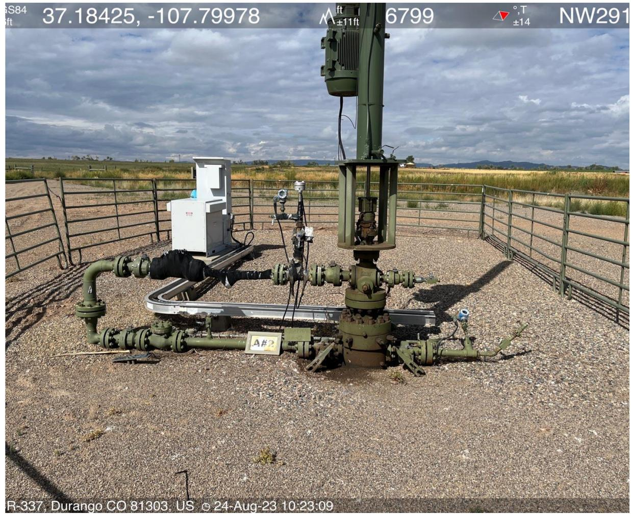
Photo #2 View of the A2 wellhead assembly.
