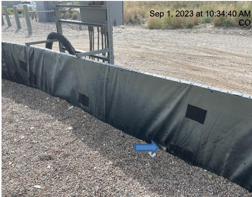
Photo # 7971 Hole in liner/liner needs maintenance
