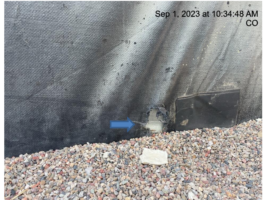
Photo # 7972 Hole in liner/liner needs maintenance
