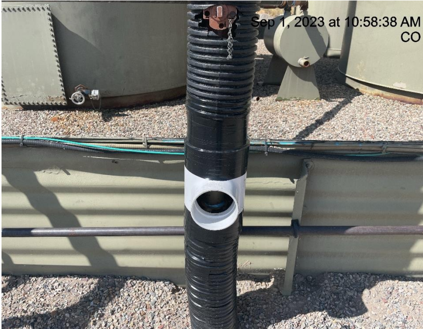
Photo # 8015 Flowline heating insulation open ended
