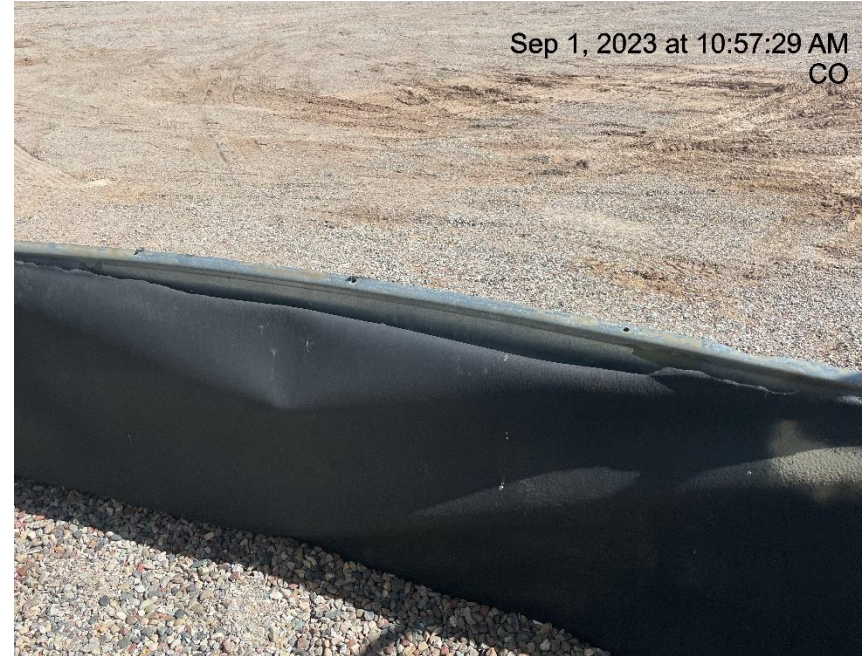
Photo # 8010 Liner needs maintenance
