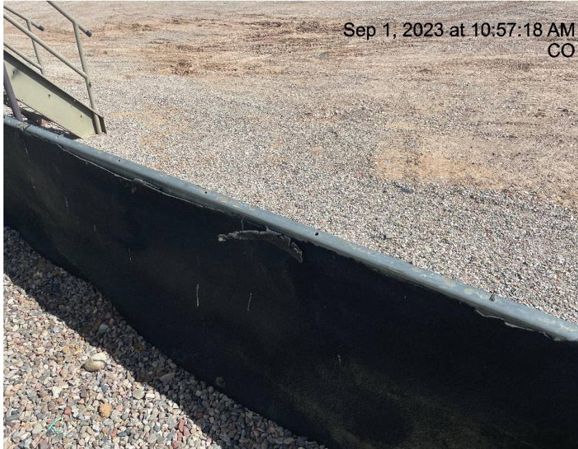
Photo # 8009 Liner needs maintenance
