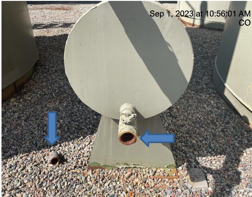
Photo # 8005 Debris & open ended load line
