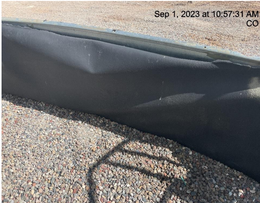
Photo # 8011 Liner needs maintenance
