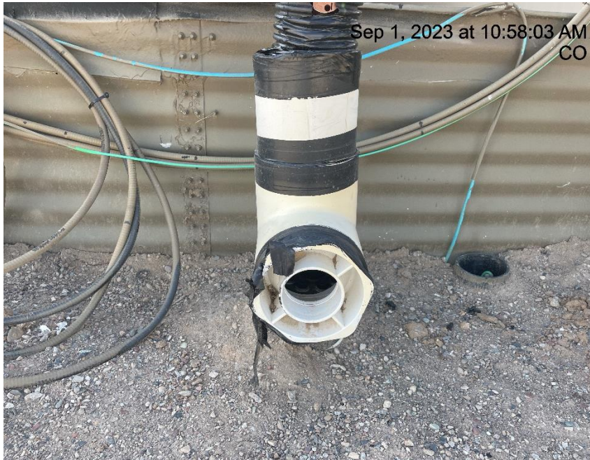
Photo # 8013 Flowline heating insulation open ended
