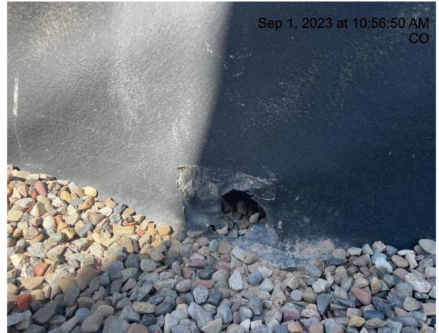
Photo # 8008 Hole in liner/liner needs maintenance
