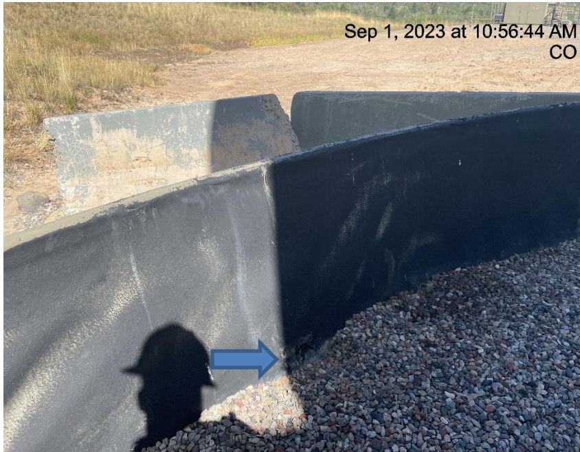
Photo # 8007 Hole in liner/liner needs maintenance
