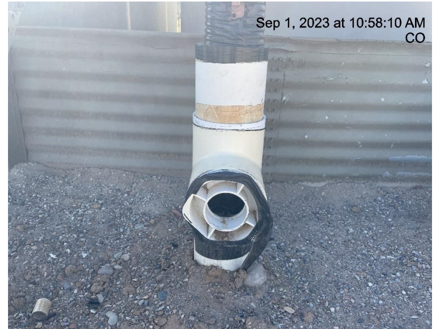
Photo # 8014 Flowline heating insulation open ended
